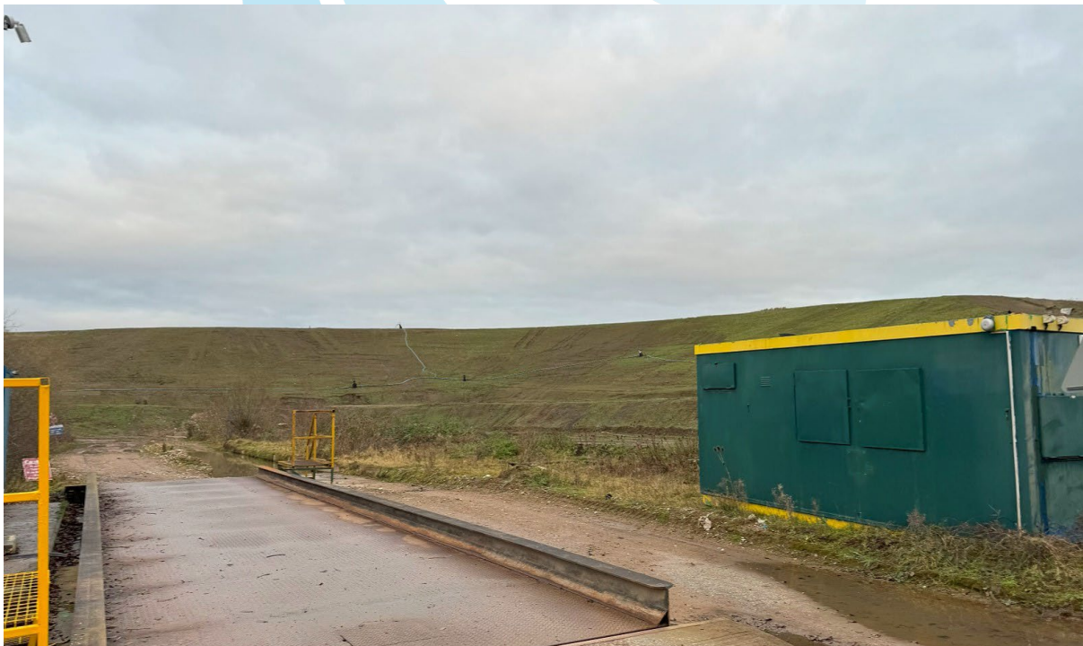
Photo 7-2 Daneshill Landfill Pre-Settlement Profile
