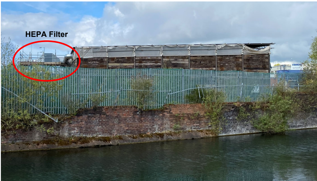
Figure 1. Asbestos Building and HEPA filter, Horseley Fields
