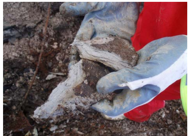
Photo courtesy of Hydrock. Plate 24. Close-up of degraded AIB/fibrous board in excavated made ground.
