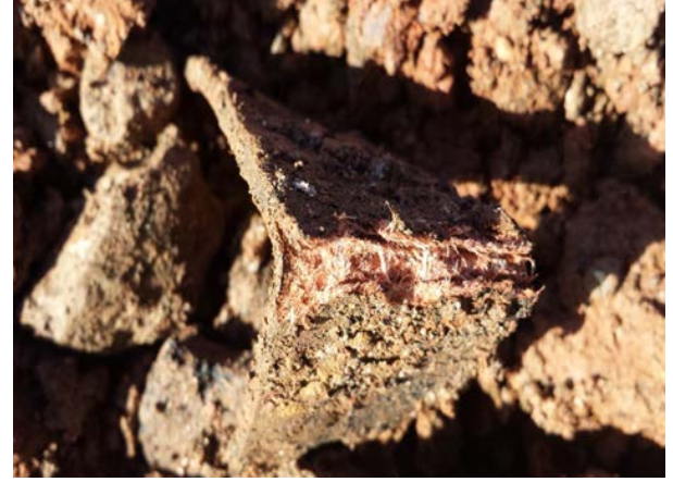
Photo courtesy of Hydrock. Plate 14. Close-up of weathered CAF gasket in excavated made ground.
