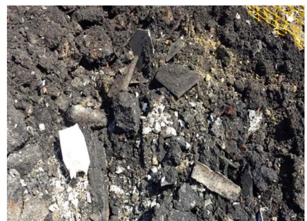
Photo courtesy of Hydrock. Plate 12. Close-up of weathered asbestos cement fragments in made ground.
