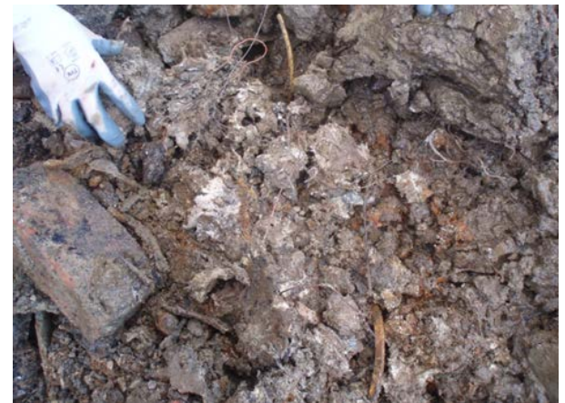
Photo courtesy of Hydrock. Plate 34. Highly degraded/disaggregated asbestos insulation/fibrous debris in excavated made ground.
