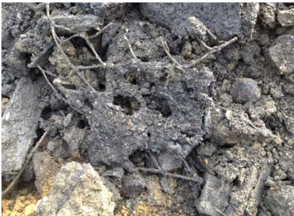
Photo courtesy of Hydrock. Plate 33. Highly degraded/disaggregated asbestos insulation/fibrous debris in excavated made ground.
