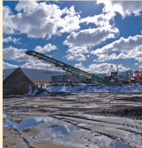
Processing plant | John F Hunt
