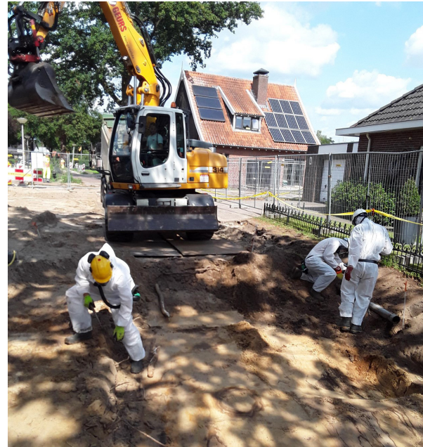
Removing asbestos contaminated soil | NTP
