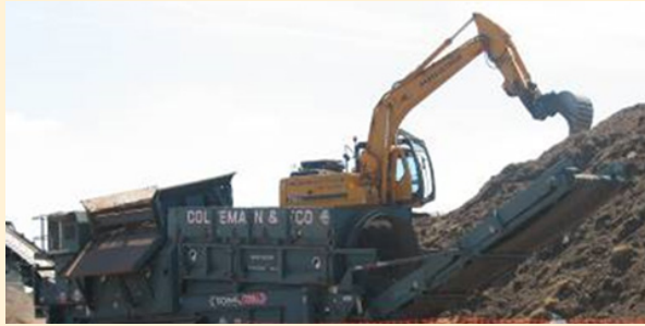
Processing plant | Ramboll
