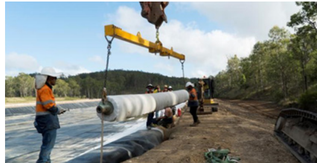
Installation of surface barrier geotextile | Curtis Barrier Intl
