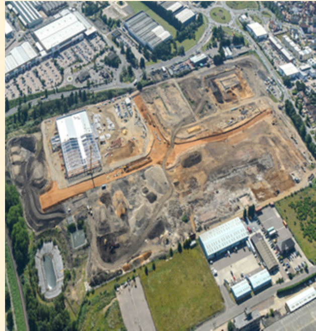
Futura Business Park – Ipswich, UK | John F Hunt
