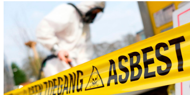
Signing of an asbestos impacted area | NTP
