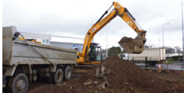
Typical remediation earthworks activities in UK | AECOM
