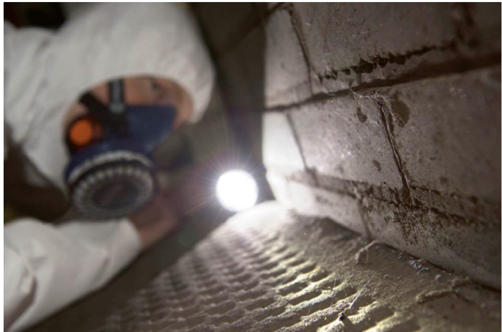
Figure 6.2 Analyst carrying out a detailed visual inspection
