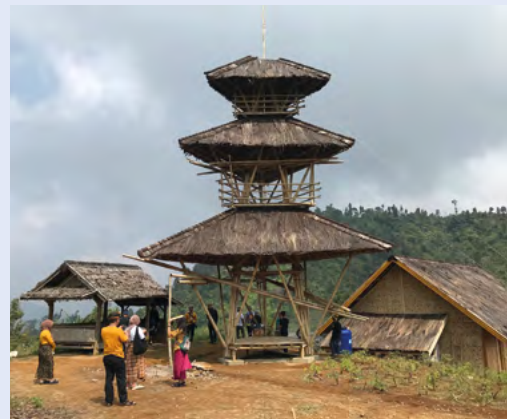
A bamboo local telecoms tower for rural Internet access in Ciptagelar, Indonesia
