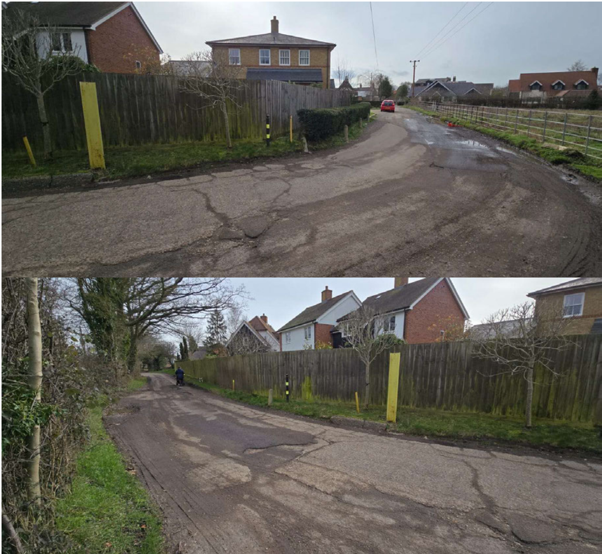
Photo 3 & 4 – Second Section of Mill Lane.
