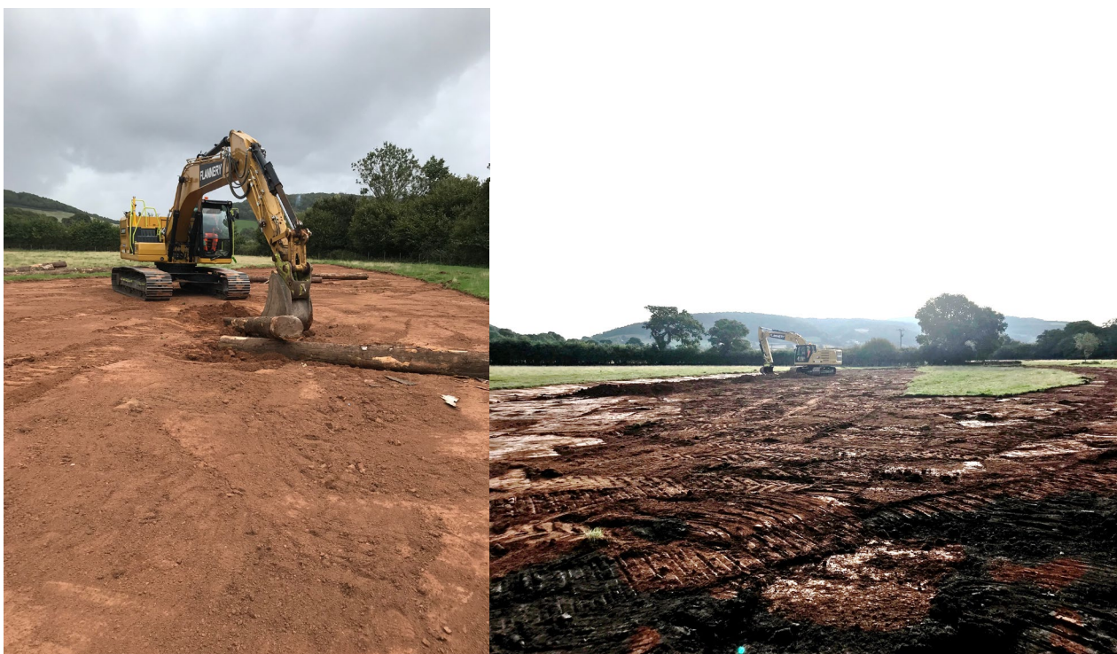
Figure 7. 1 Photographs of construction.
