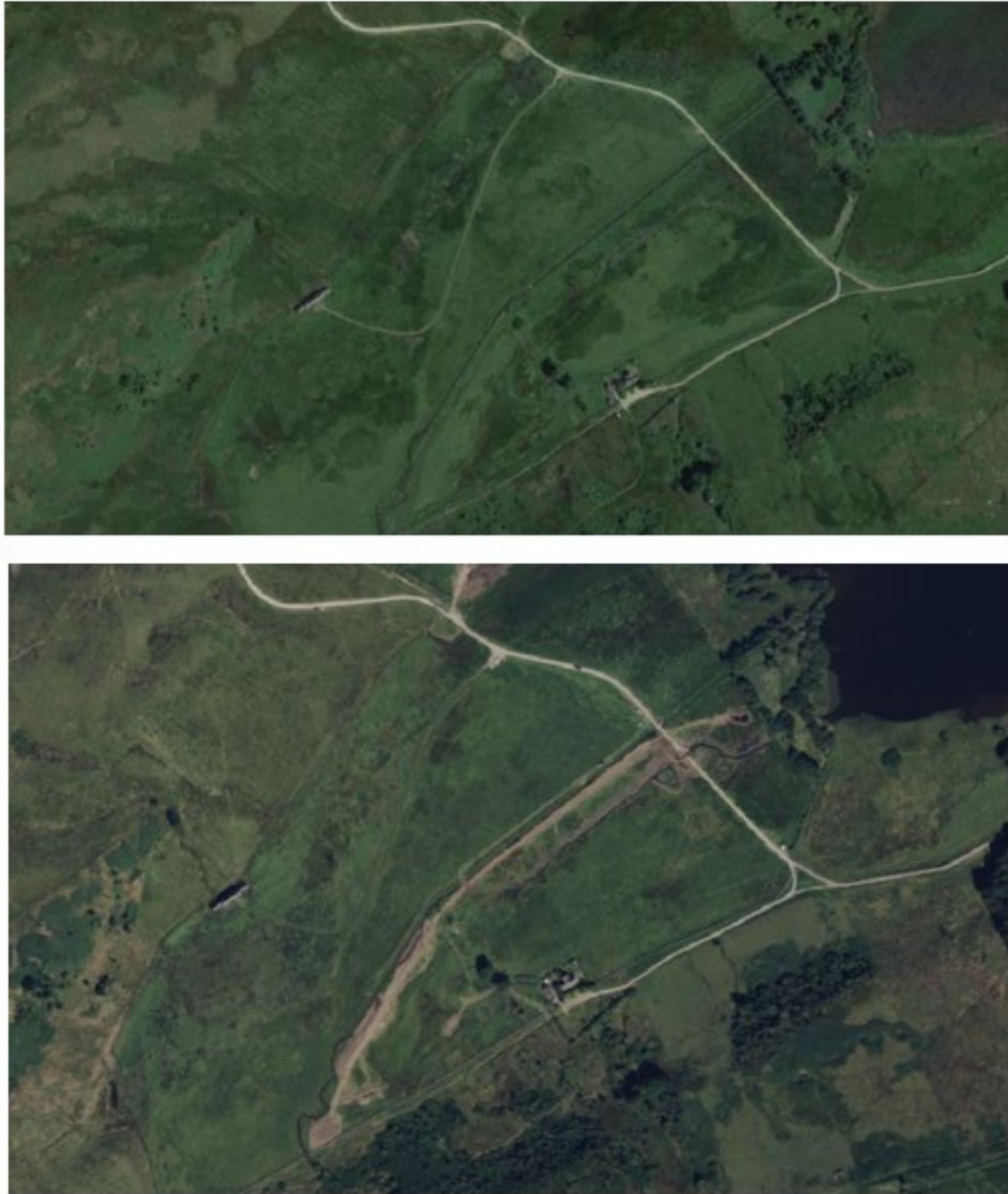
Figure 11.1 Aerial Photographs of pre-construction (top) and post-construction (bottom).
