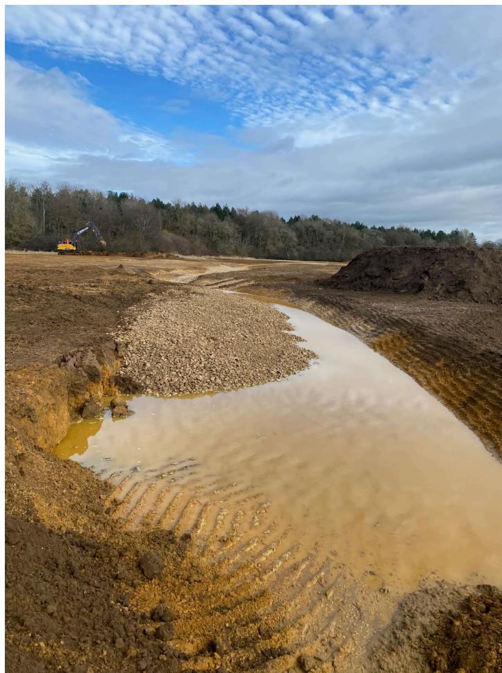
Figure 12.2 Photographs of pre-construction (top) and during-construction (bottom).
