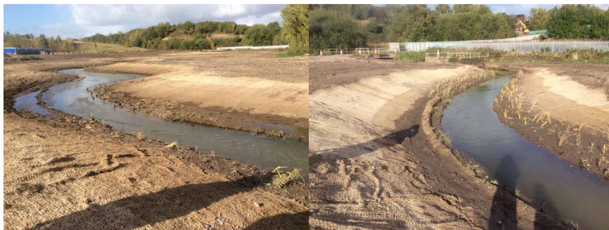
Figure 8.1 Photographs taken during the construction phase.
