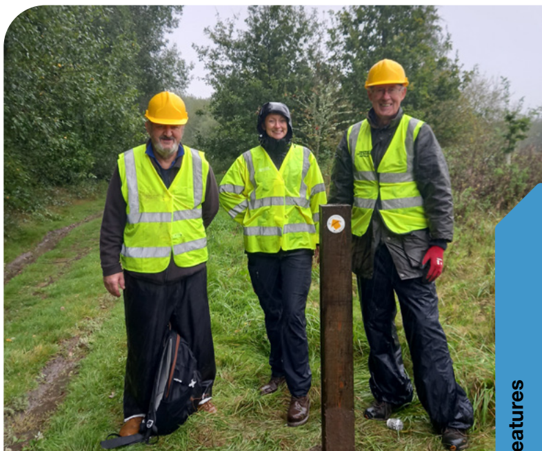
Installing a waymarker at Borden © Hampshire Ranger Service
