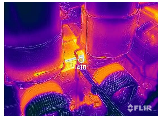
Figure 1: MAIB observed hot surface exceeding 220°C
