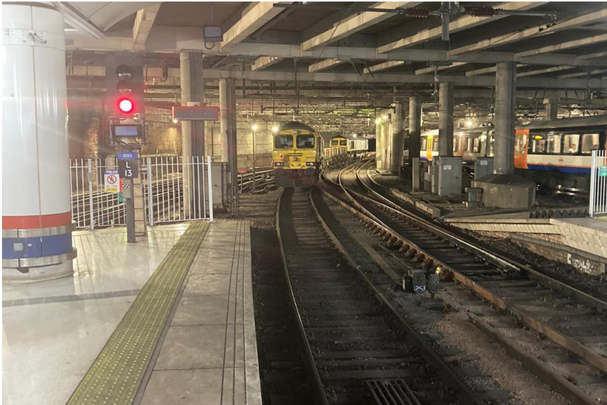
The engineering train post-incident, stopped in the throat of the station (courtesy of Network Rail).
