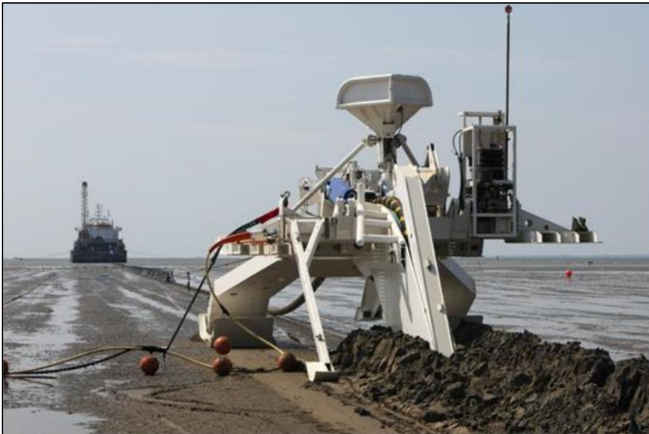
Figure 3.18: Photo Of Typical Power Cable Plough (Photo Credit: Boskalis)
