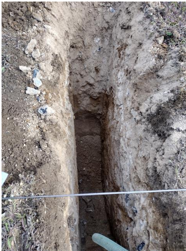
Photo 2 – Example of Ground conditions in SA04
