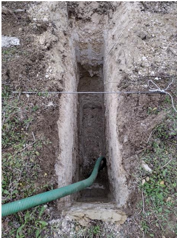
Photo 1 – Example of Ground conditions in SA02
