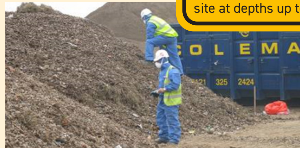
Asbestos finds—hand picking | Ramboll
