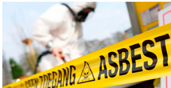
Signing of an asbestos impacted area | NTP
