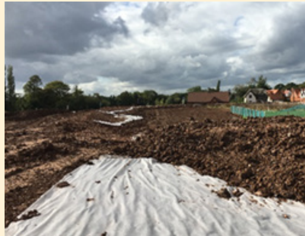
Installation of the cover system | AECOM
