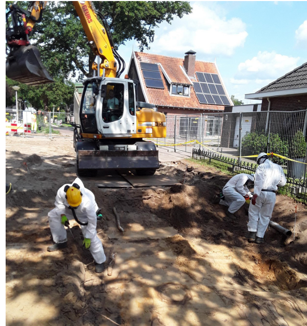
Removing asbestos contaminated soil | NTP
