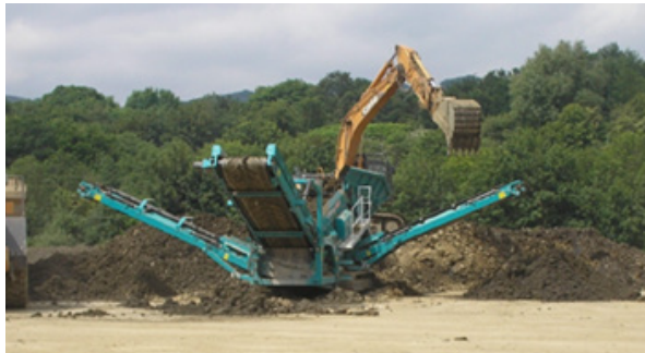
Mechanical screening of excavated soil | AECOM
