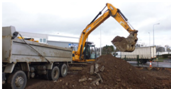
Typical remediation earthworks activities in UK | AECOM
