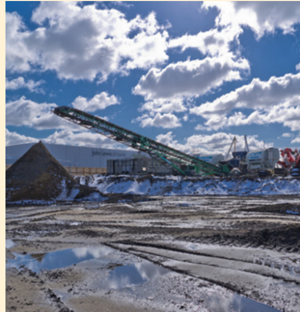
Processing plant | John F Hunt
