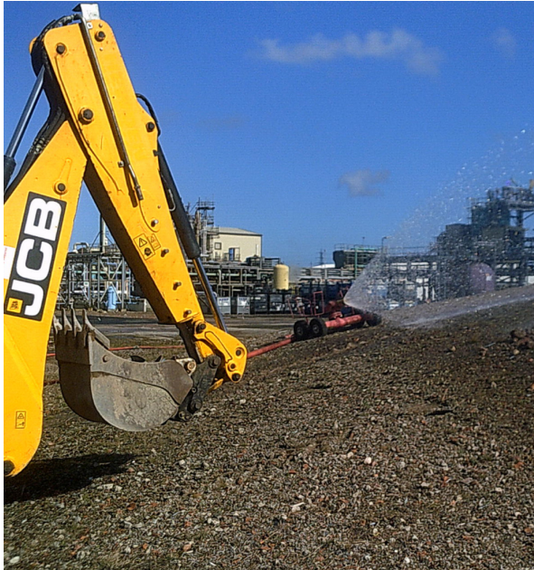
Damping down of stockpiled material with water spray | AECOM
