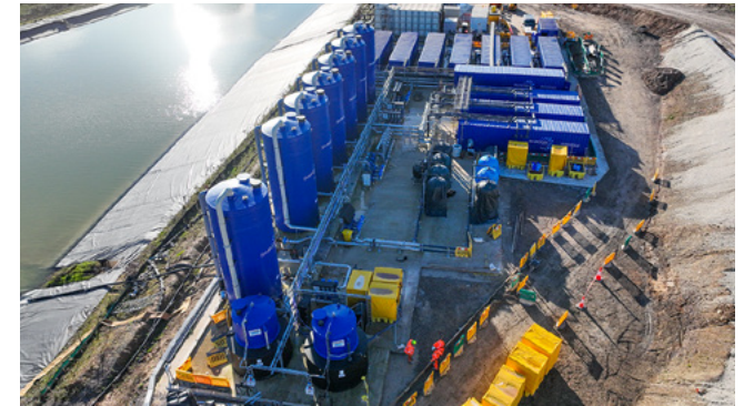
The facility at the tunnel's south portal site.
