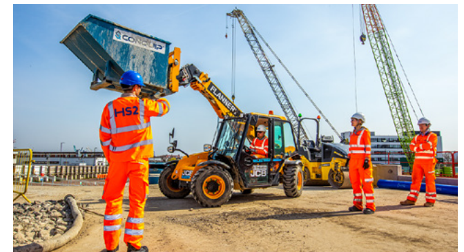
An electric digger at HS2's Victoria Road site in west London.
