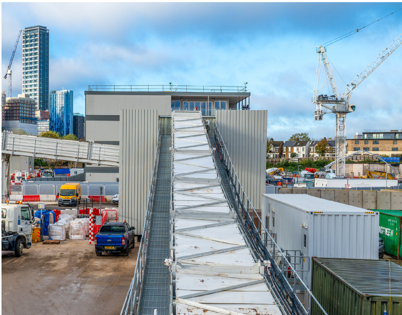
The conveyor at Old Oak Common.
