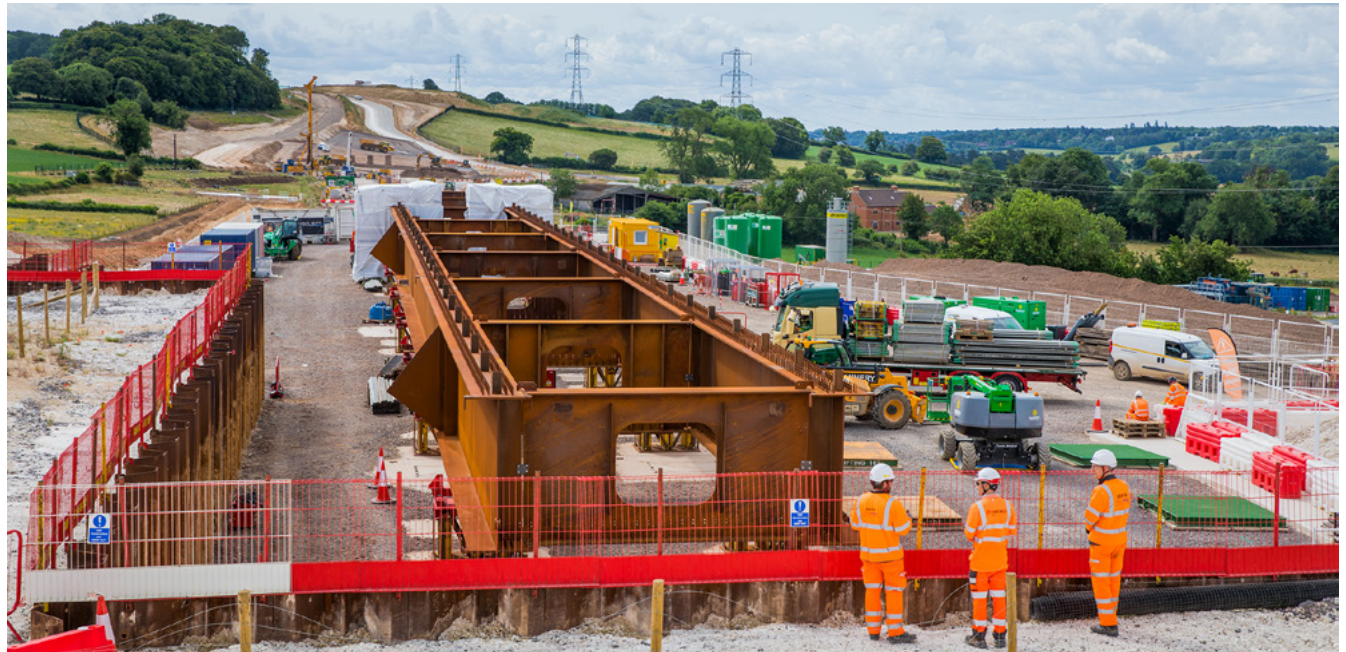
Construction progress on the Wendover Dean viaduct.
