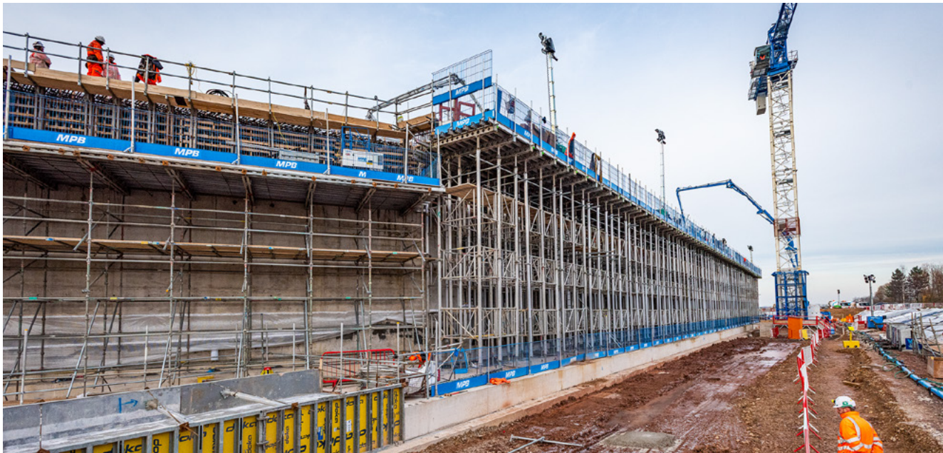
Construction of the Marston box bridge.
