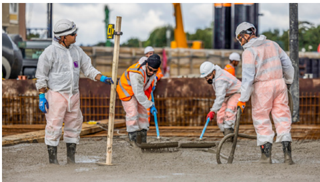
UK's largest pour of environmentally-friendly concrete in London.
