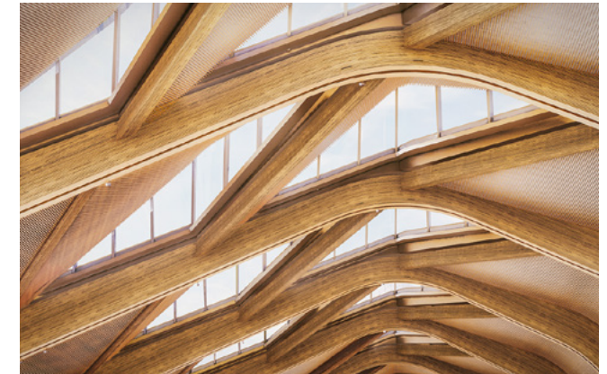
Roof detail at Interchange station.
