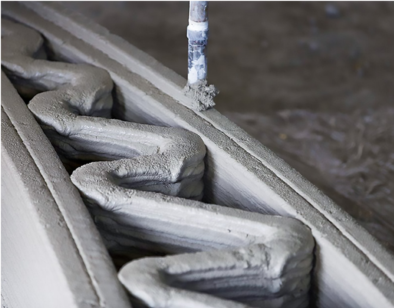
The 3D concrete printing system in action.
