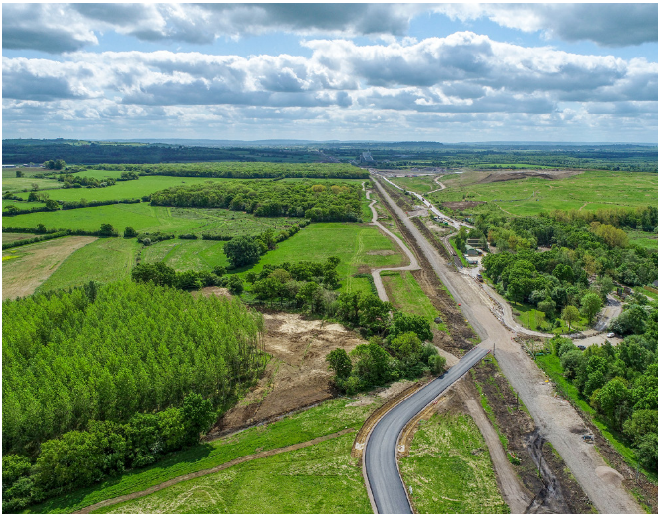
An aerial view of the temporary access road.
