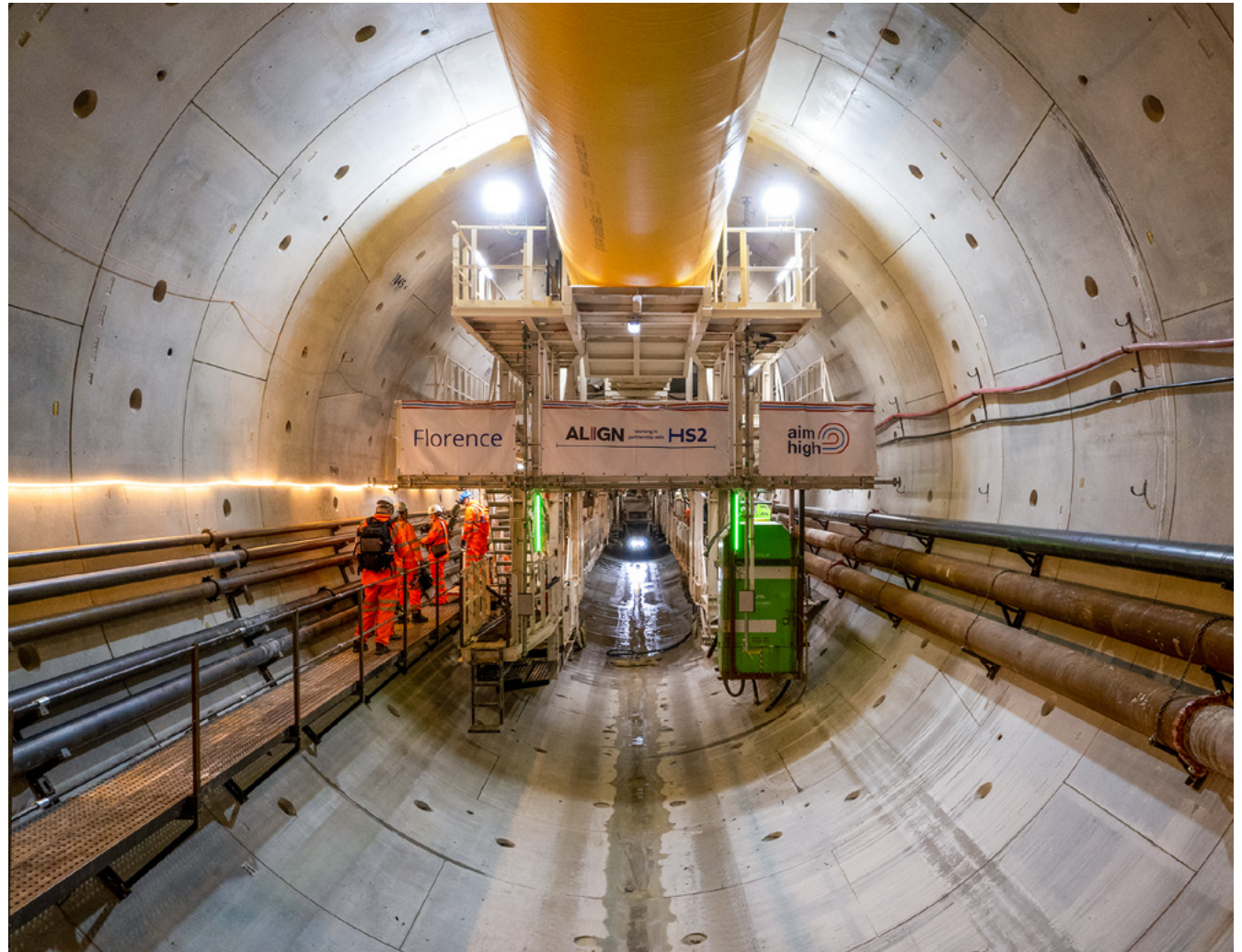
Tunnelling machine Florence in the Chiltern tunnel.
