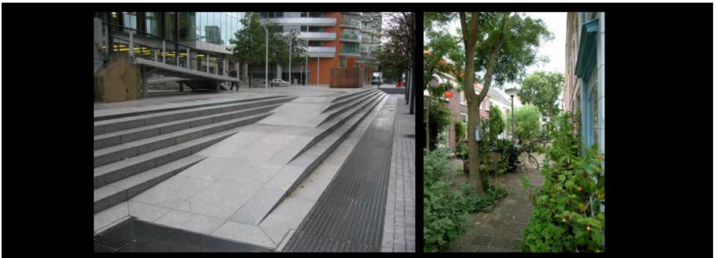
(right) Wheelchair and pushchair ramp incorporated with steps, Paddington Basin, London Image
