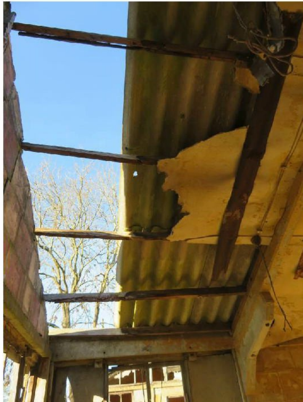
Photograph 10: Purlins at regular centres to support roof covering and internal finishes
