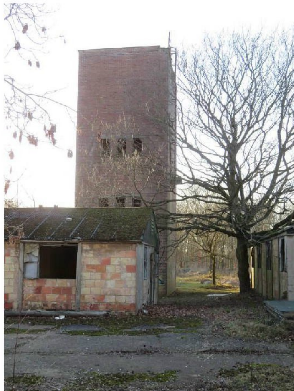
Photograph 24: Water tower east facing elevation
