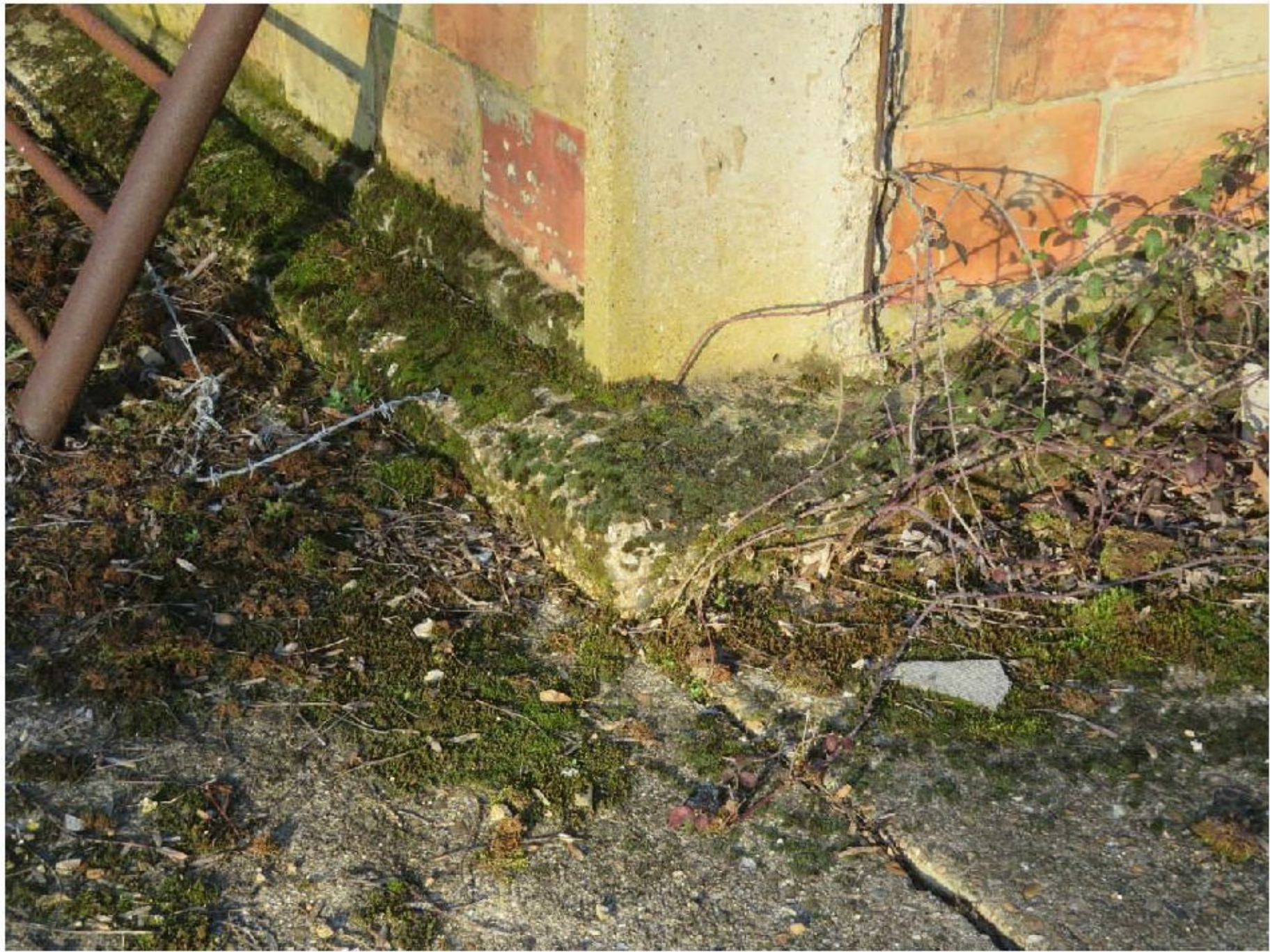
Photograph 23: Projection at ground possibly suggesting concrete raft foundation
