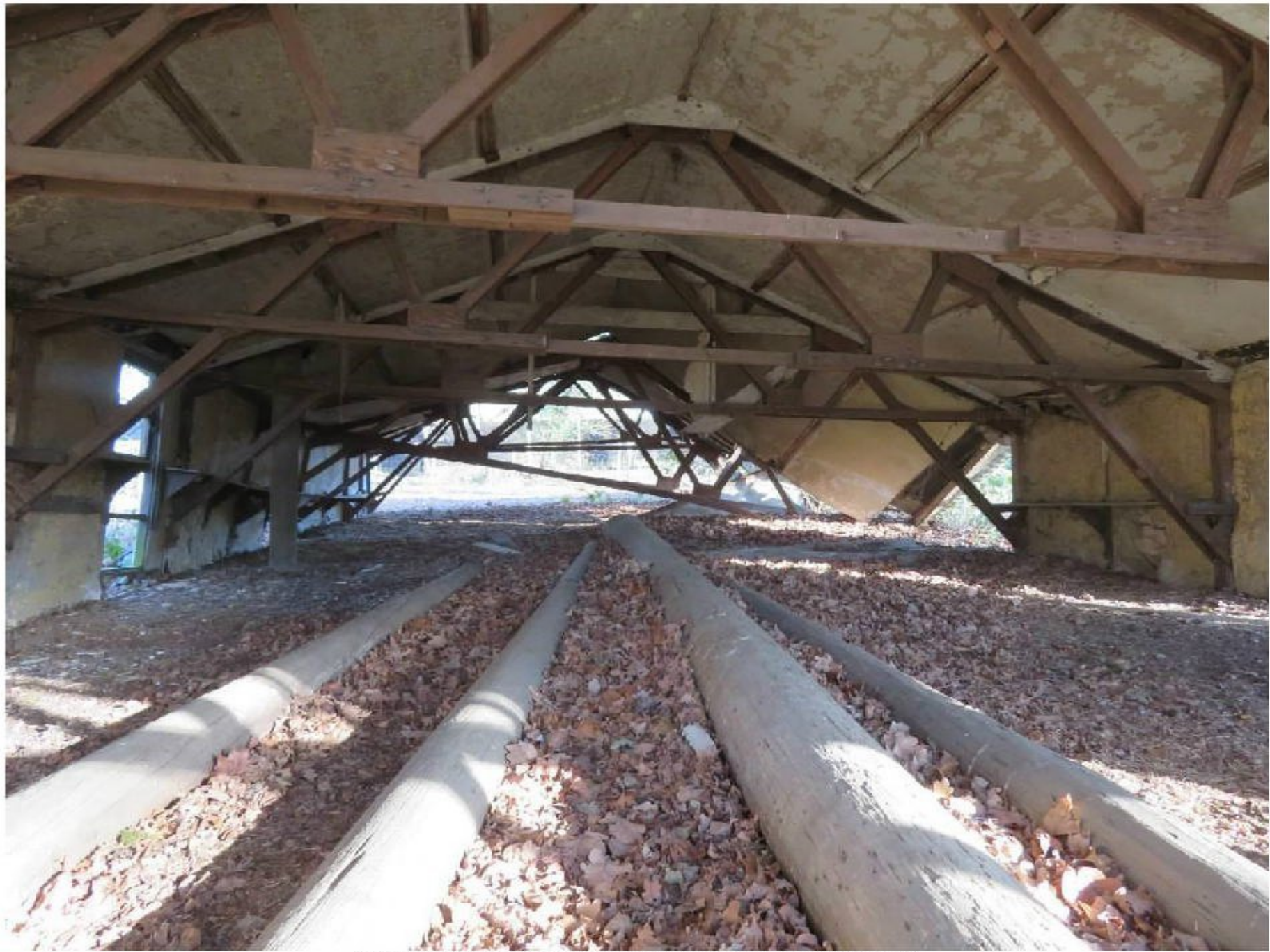
Photograph 15: Roof trusses to Building 8
