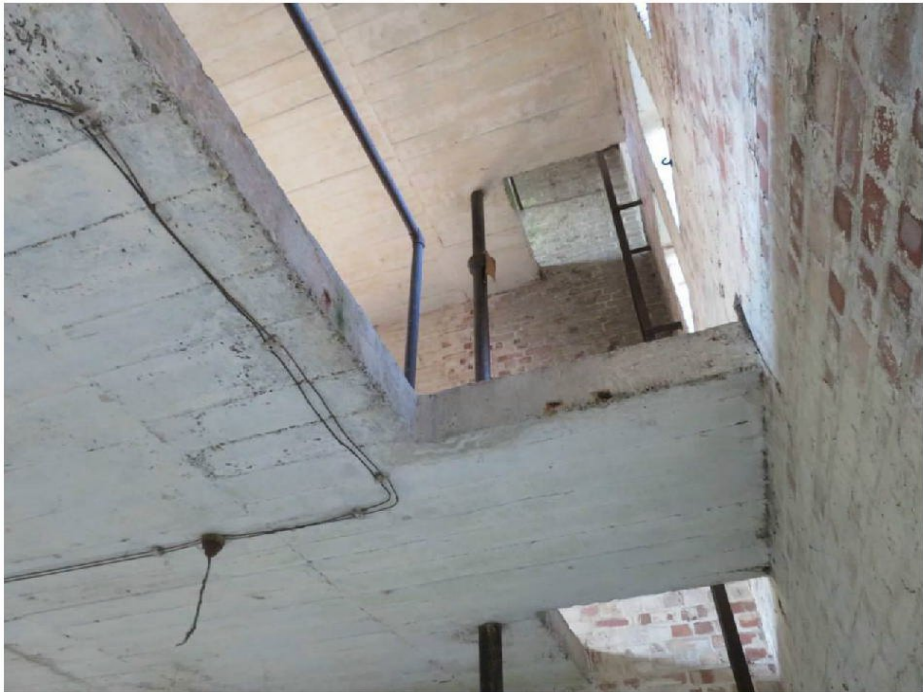
Photograph 17: Internal concrete floors to Water Tower
