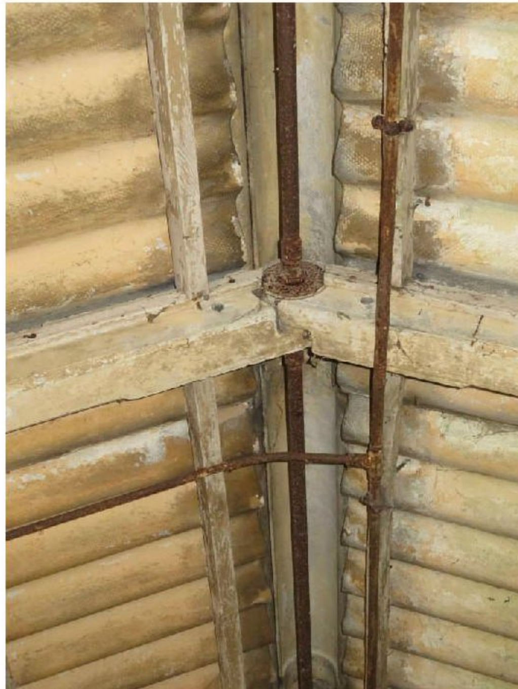
Photograph 6: Ridge tie with patten plates either side of frame
