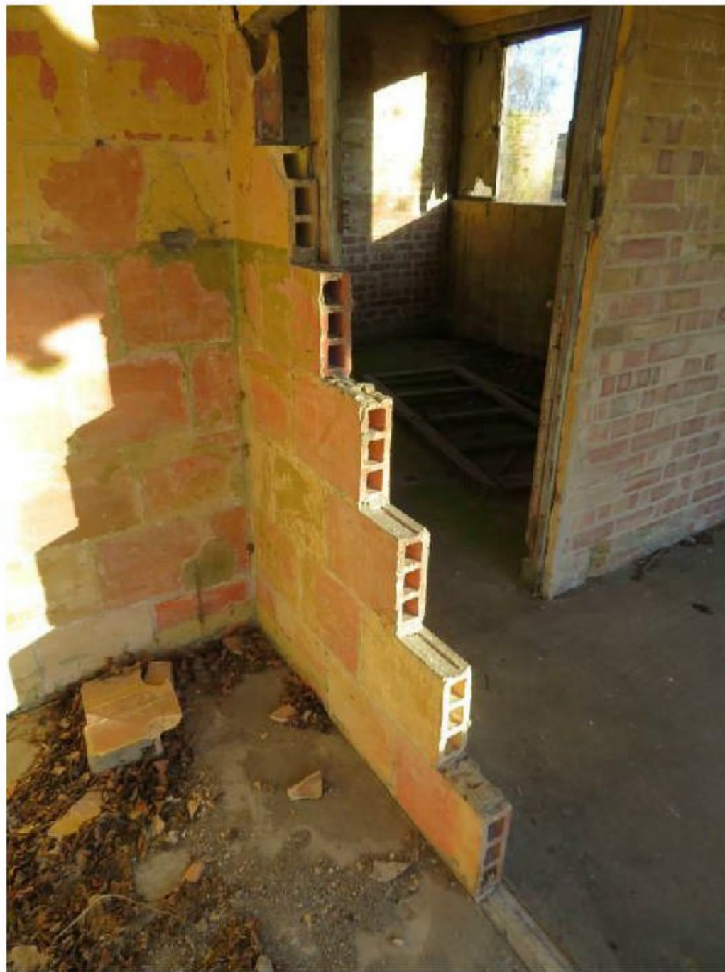
Photograph 7: Hollow blocks used as infill and some intermediate walls
