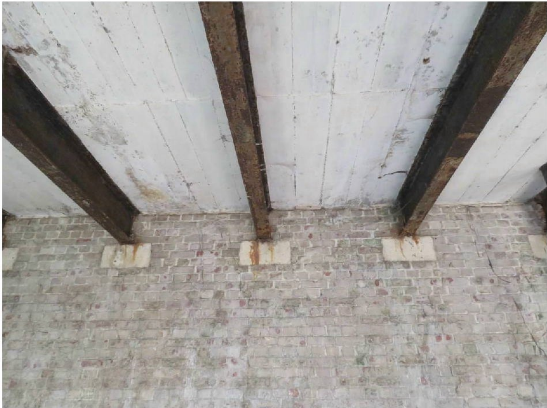
Photograph 28: Steel beams below water tank level with concrete floor over
