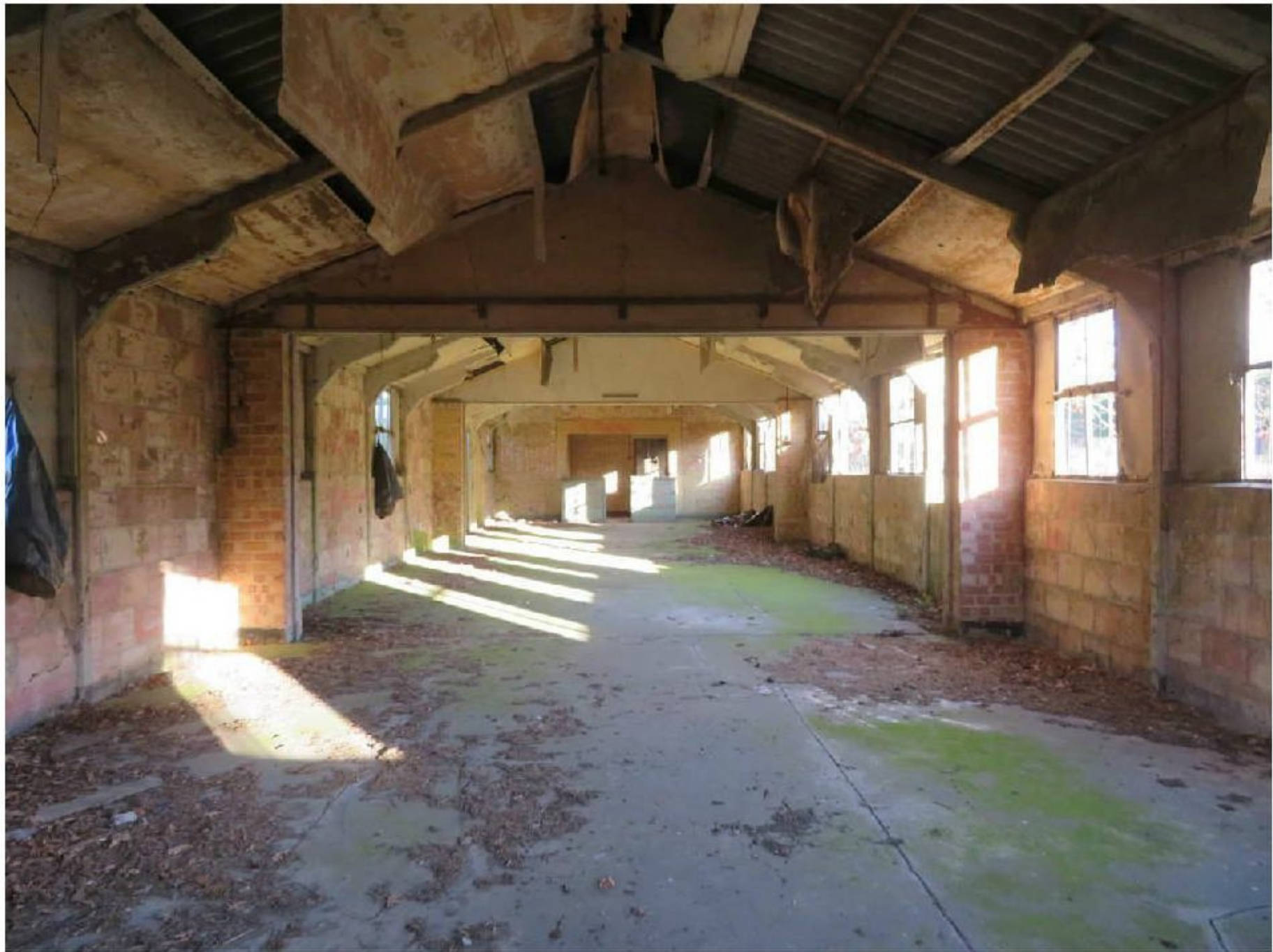
Photograph 13: Concrete floor in Building 3
