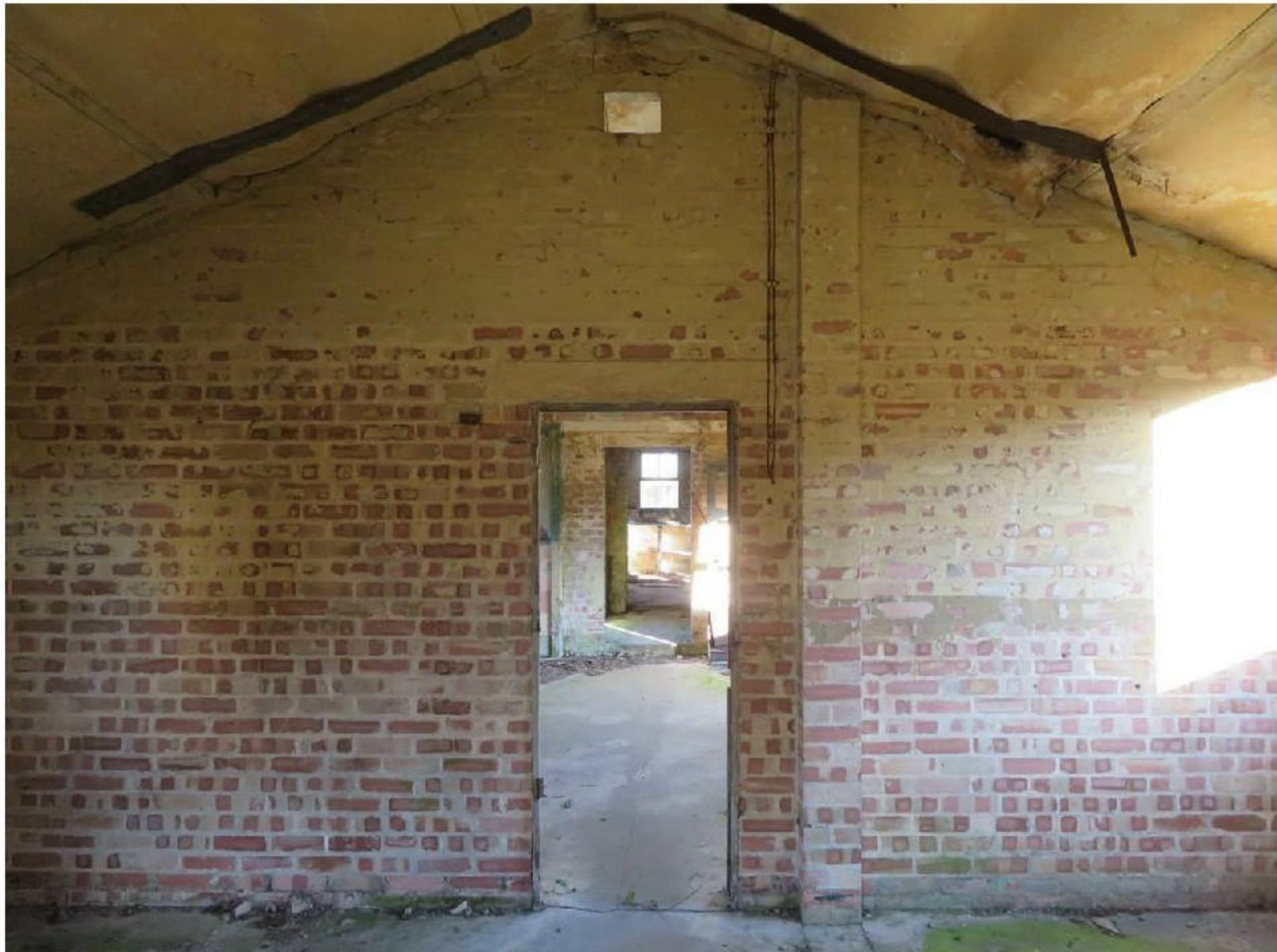
Photograph 12: Internal cross wall in brick with thickening pier
