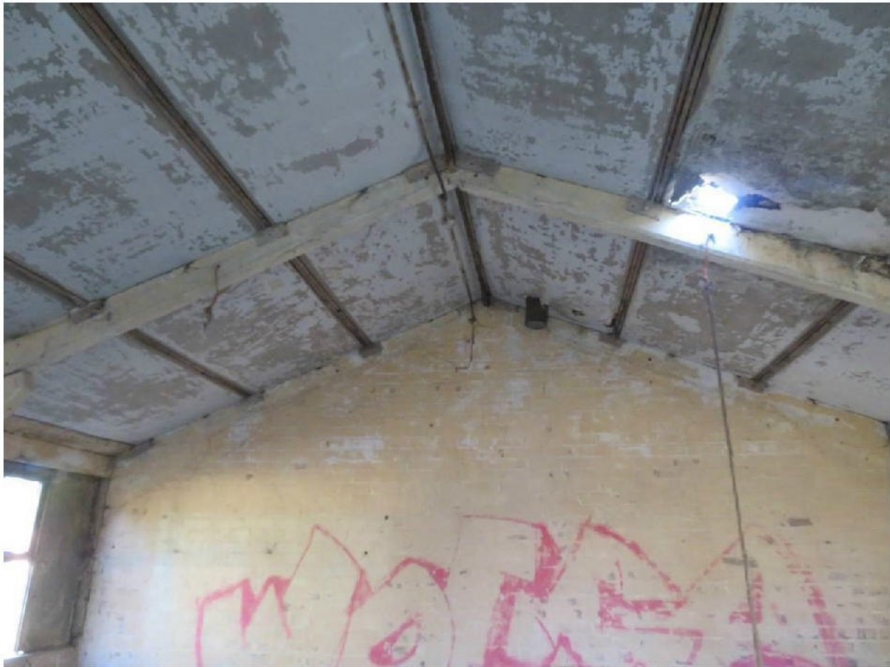
Photograph 11: Roof with internal plasterboard between purlins
