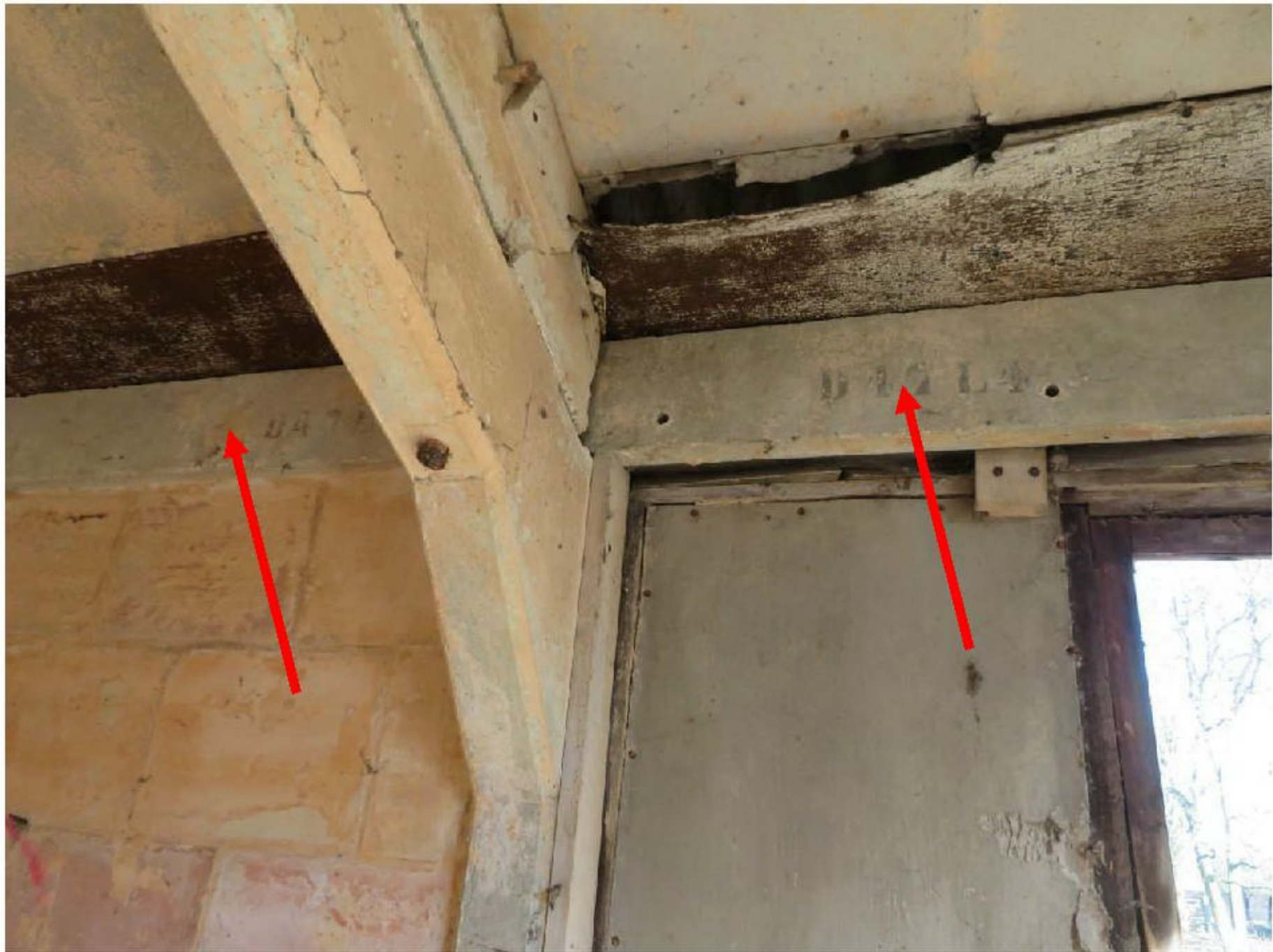
Photograph 3: Pre-cast concrete eaves plates
