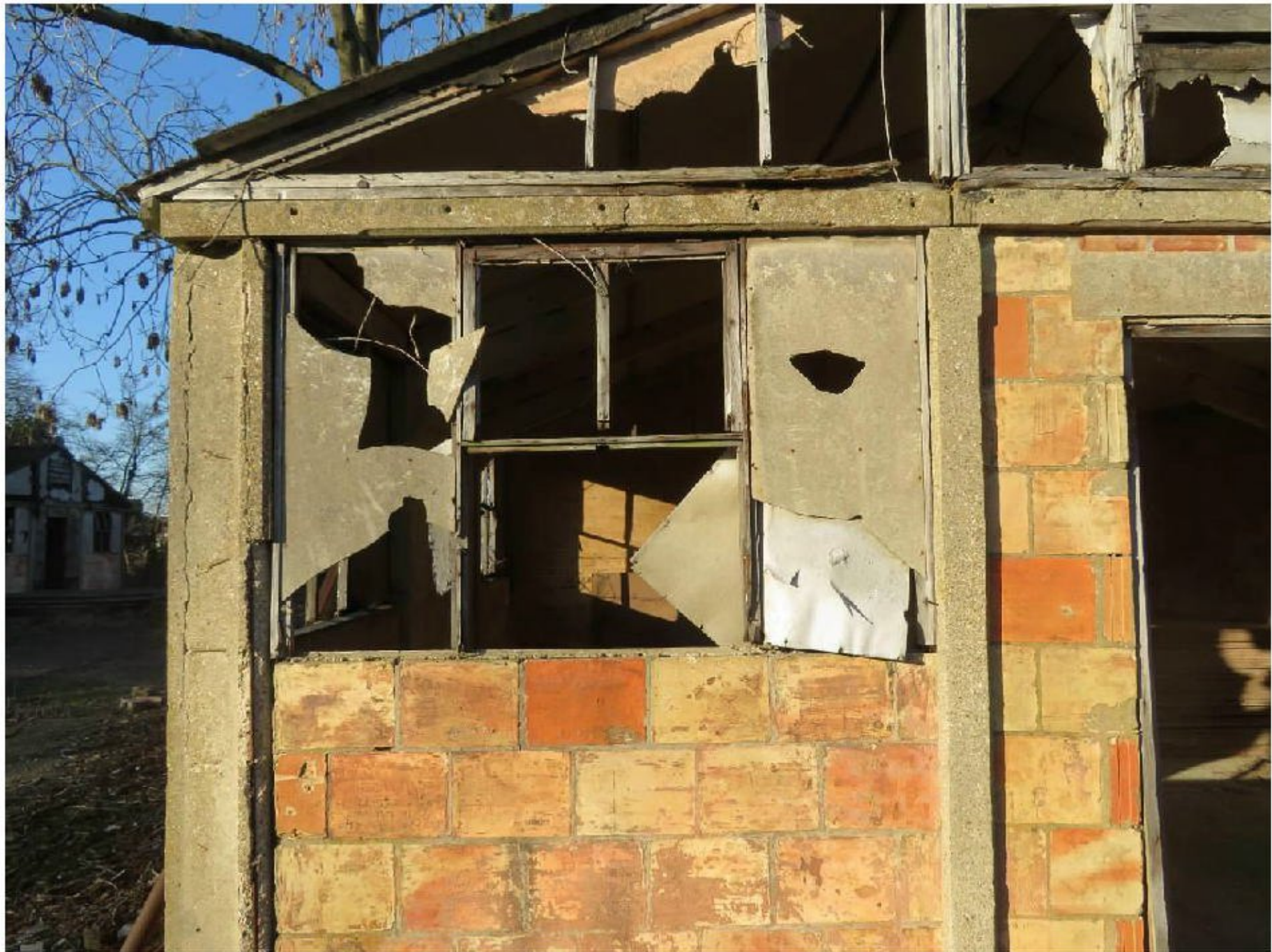
Photograph 9: Timber windows with side panels in asbestos board
