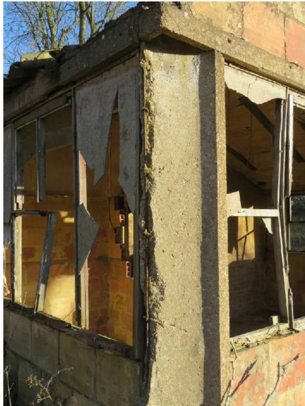
Photograph 4: Corner post with eaves plates above
