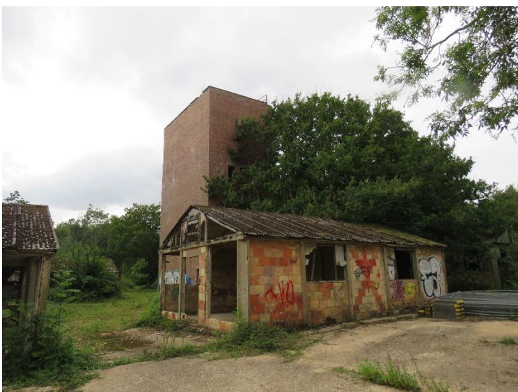
Figure 7. Buildings on the southern part of the Site.
