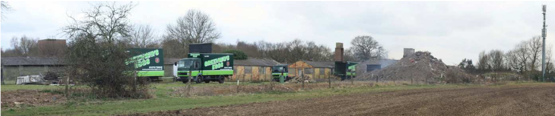
Figure 2: Existing view towards site from open countryside
