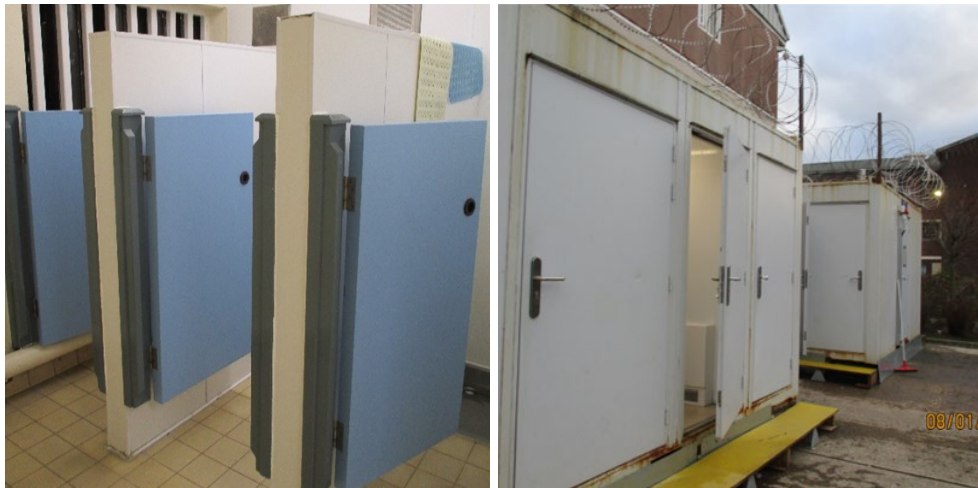
G wing showers (left) and temporary shower block outside A wing (right)
