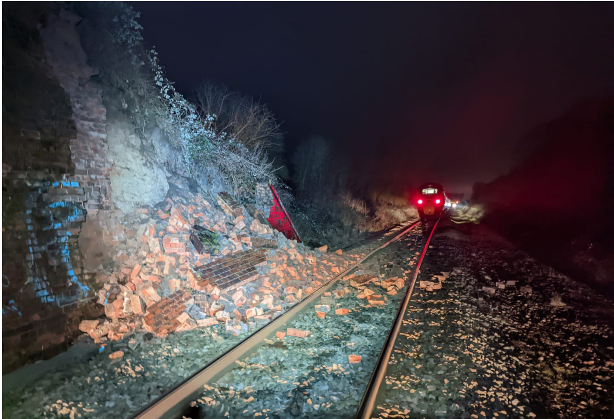
Figure 2: Debris and rear of stationary train soon after the accident (courtesy of Network Rail).
