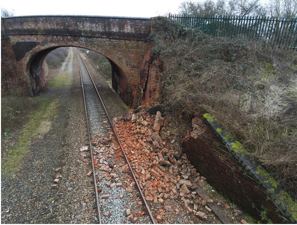
Figures 6a and 6b: Collapsed south-west wing wall on 11 February 2023.
