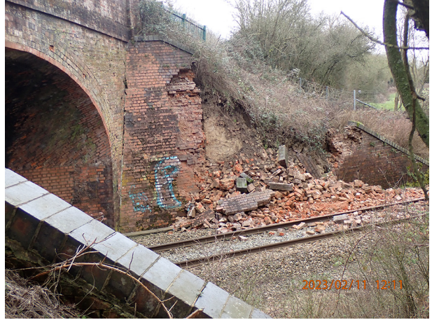
Figures 6a and 6b: Collapsed south-west wing wall on 11 February 2023.
