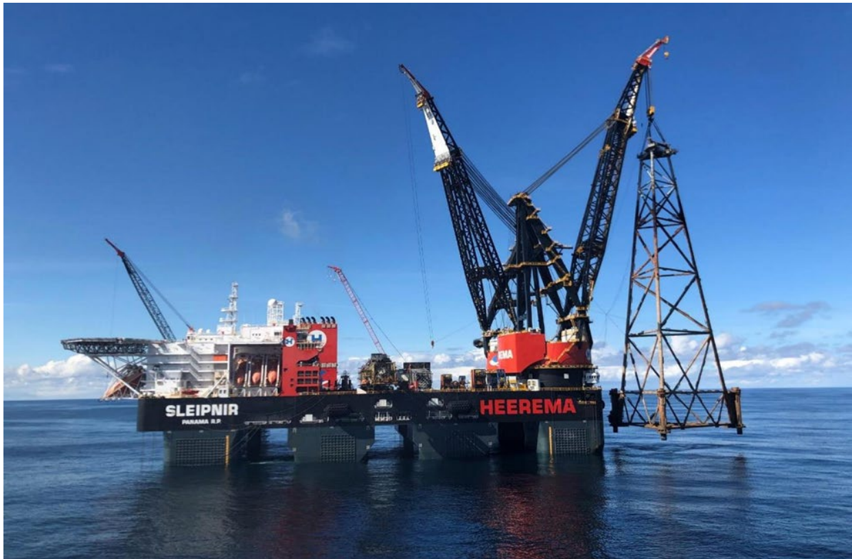
Figure 8-5: Sleipnir removing the entire flare jacket in a single lift
