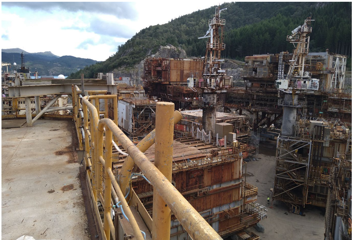
Figure 8-12: Bravo modules relocated on the quayside ready for demolition
