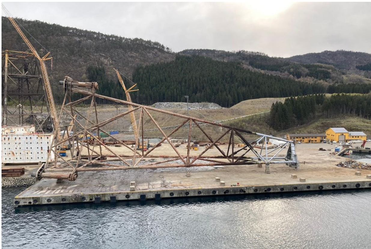
Figure 8-6: Flare jacket as it was landed on the quayside
