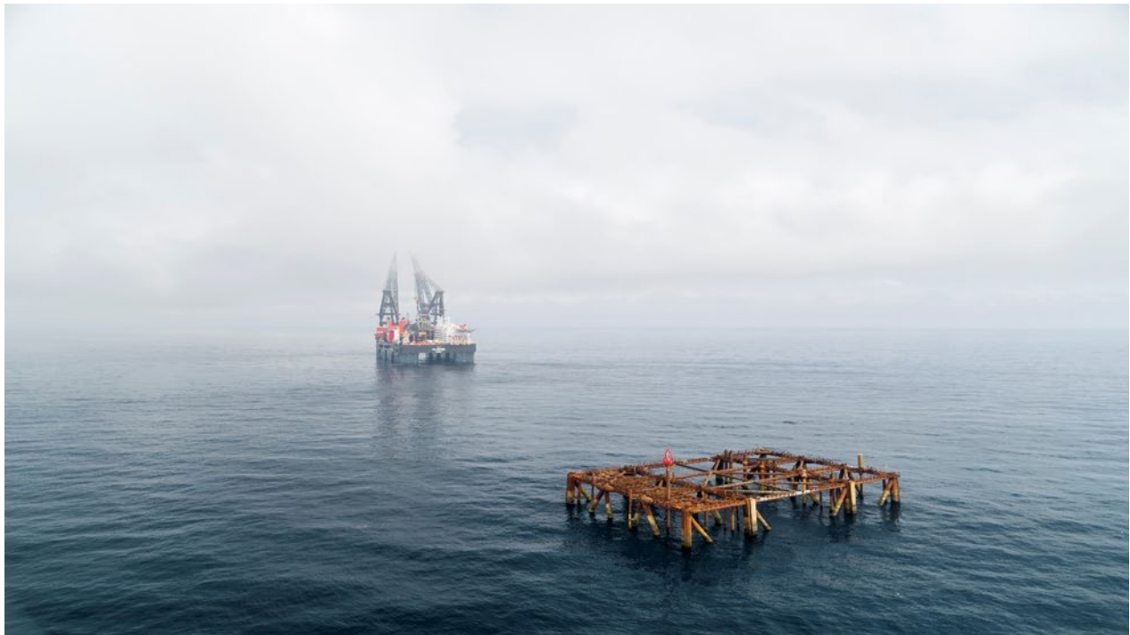
Figure 8-10: Topsides removal complete offshore
