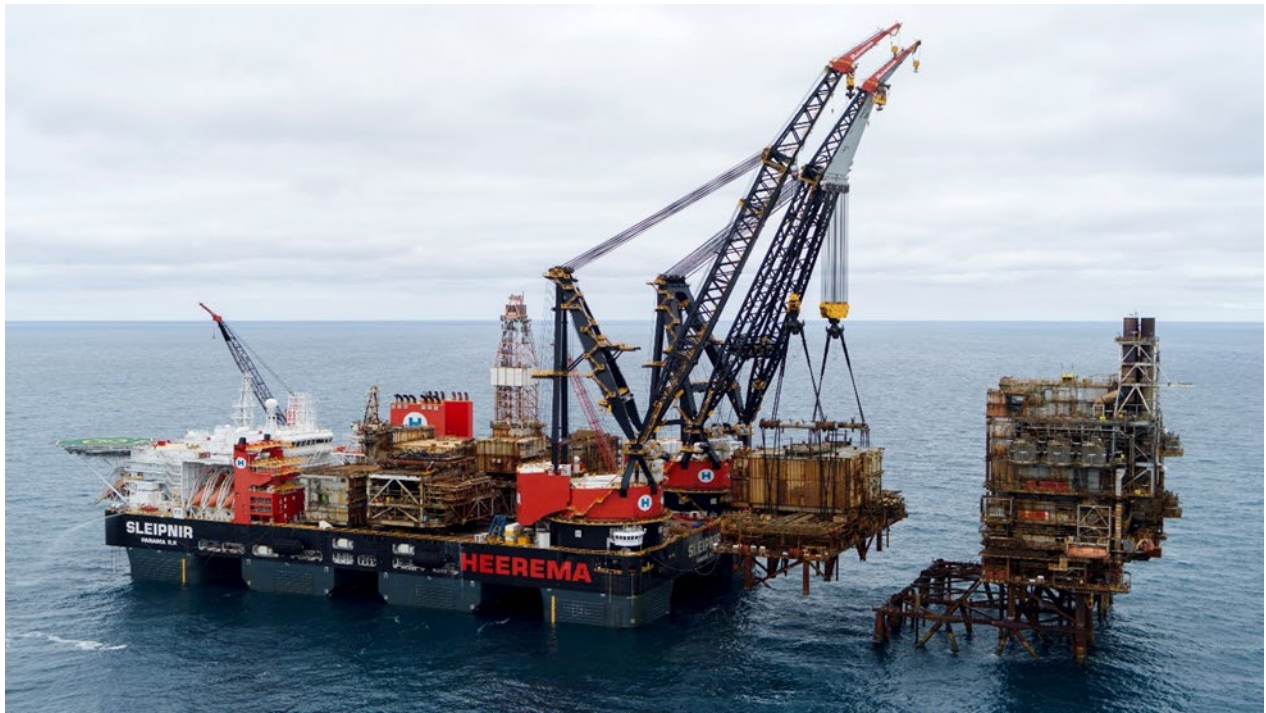
Figure 8-9: West Module Support Frame (MSF) removal
