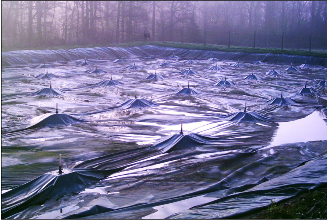
Figure 5: A floating plastic cover on an earth-banked slurry lagoon. Image credit: Defra
