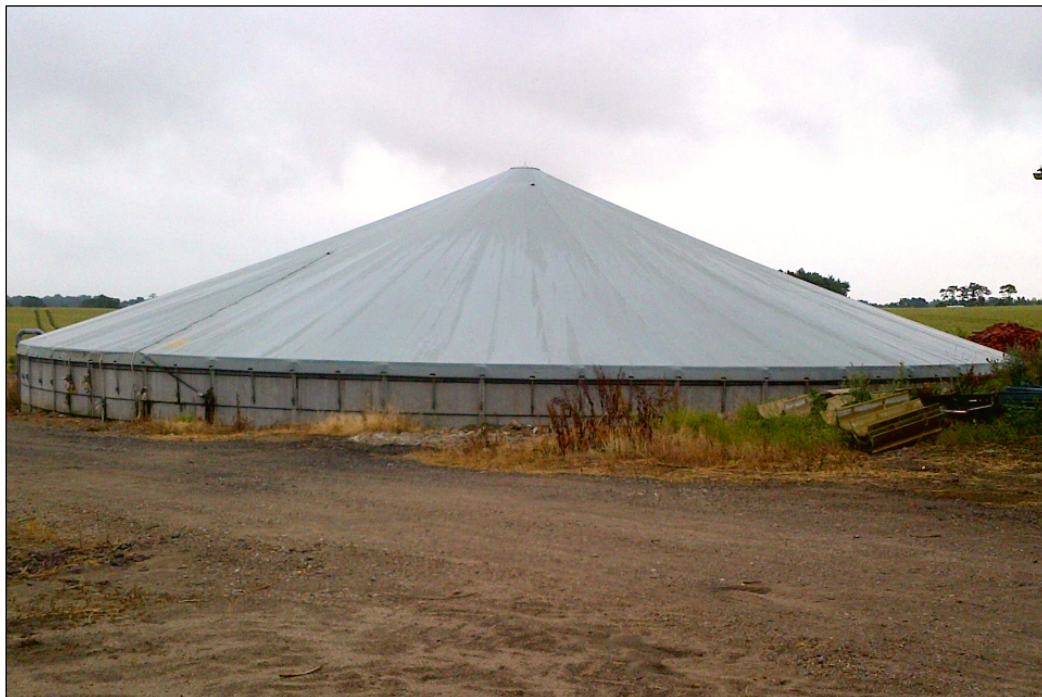
Figure 4: A fixed cover on a slurry tank.
