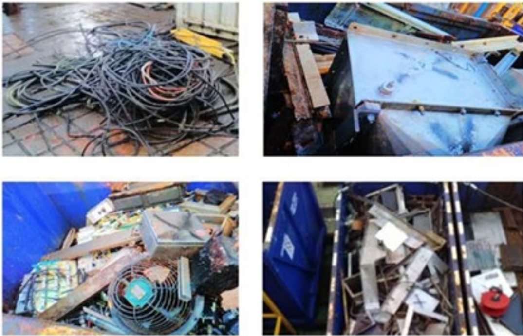
Figure 8-13: Derrick Destruct Waste Segregation (Cable, Steel & Electrical Equipment)
