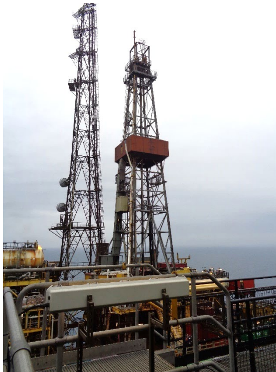
Figure 8-2: Close up of original Drilling Derrick Structure, adjacent to Telecoms Tower
