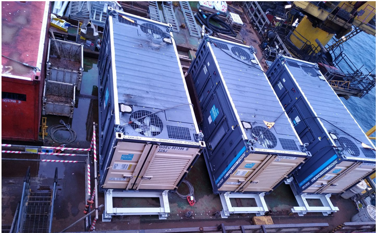
Figure 8-10: Power Generation Units Installed
