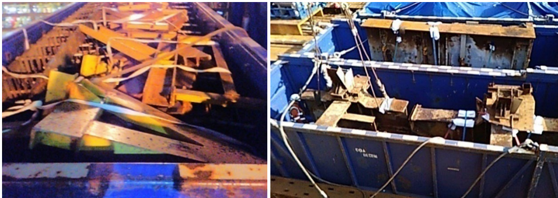
Figure 8-14: Derrick Destruct Waste Segregation (Scrap Metal)
