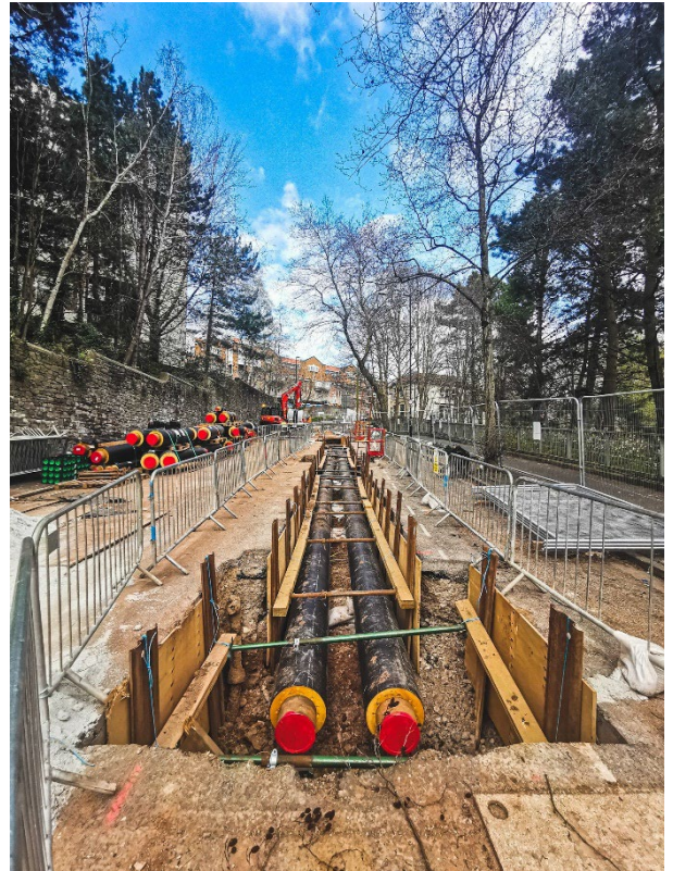
Photo credit Vital Energi
