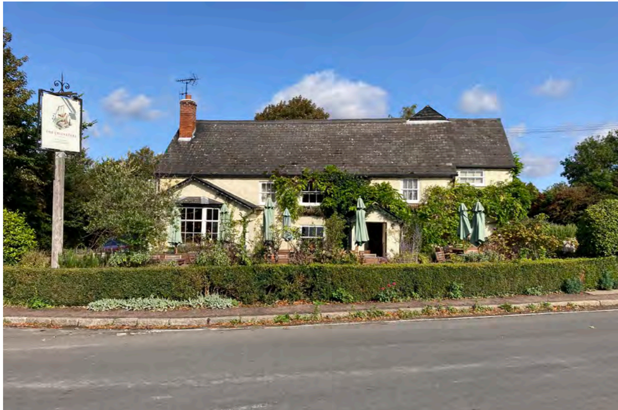
Figure 4.5. Front elevation of The Cricketers public house.
