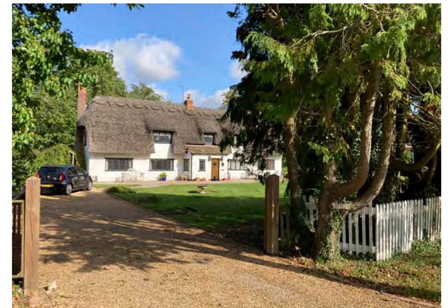
Figure 4.4. Front elevation of Lantern Thatch from front entrance.
