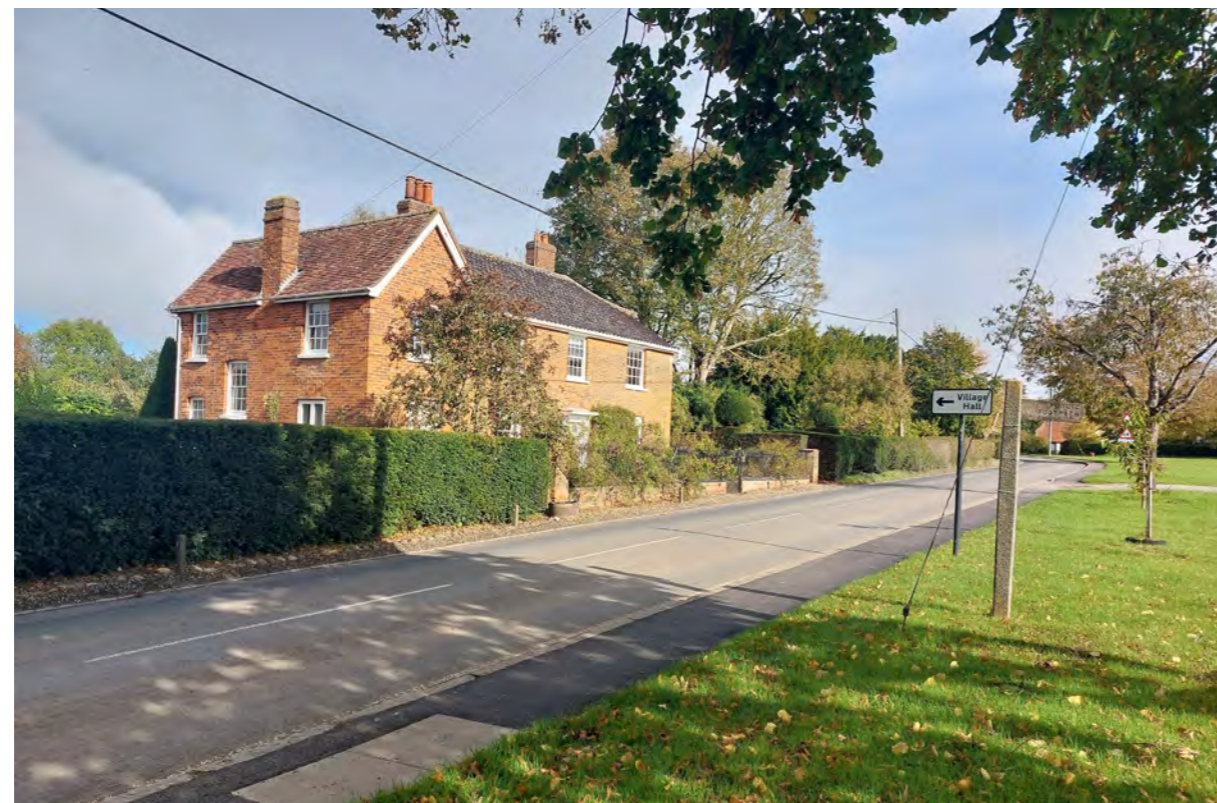
Figure 4.13. Ivy Cottage fronting the western side of the B1038.
