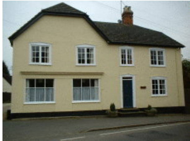
Picture 1.10 Original shopfront visible on Pavitts, High Street
