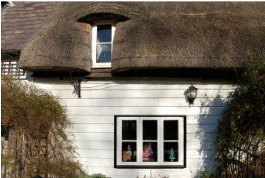
Picture 1.11 Narrow dormer and weatherboarding, cottage off Middle Street
