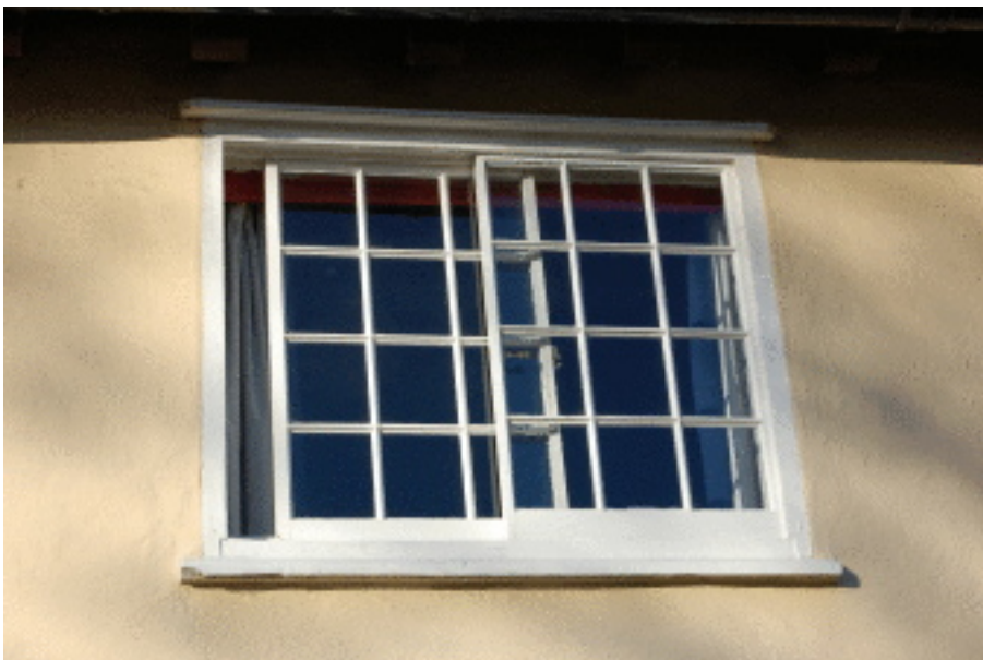
Picture 1.8 Sliding horizontal sash window on the Guildhall, Church End
