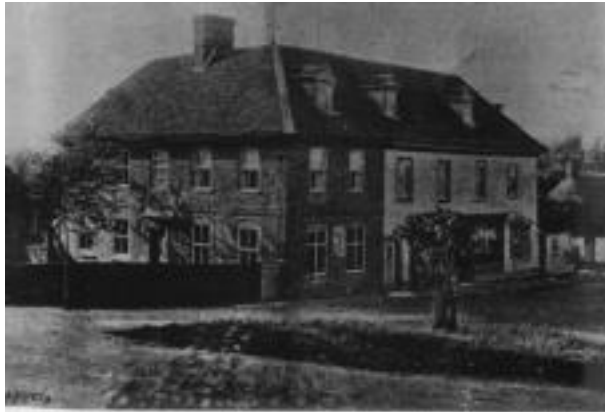
Picture 1.15 The Old House prior to 1915 showing the shopfront
