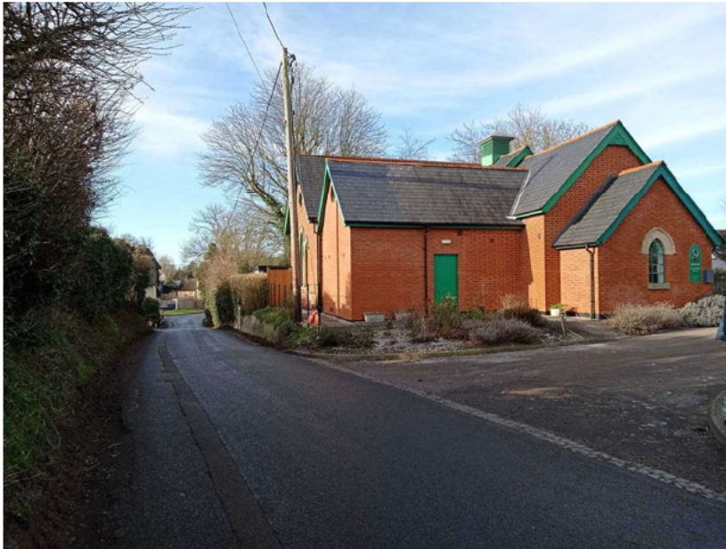
Photo 3: Village Hall in Berden looking west showing section of narrow carriageway with no footways and tight bend
