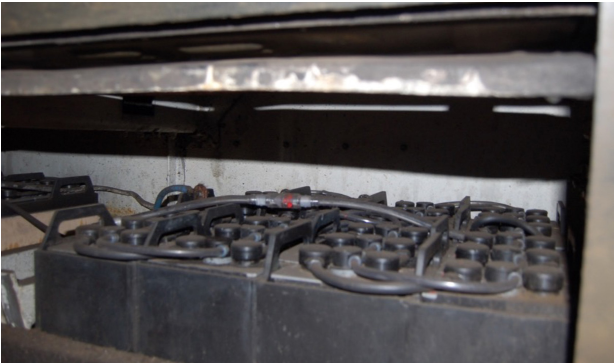
Figure 89: Arrangement of cells in the battery box of a mark 3 passenger coach (The School of Engineering of The University of Edinburgh)
