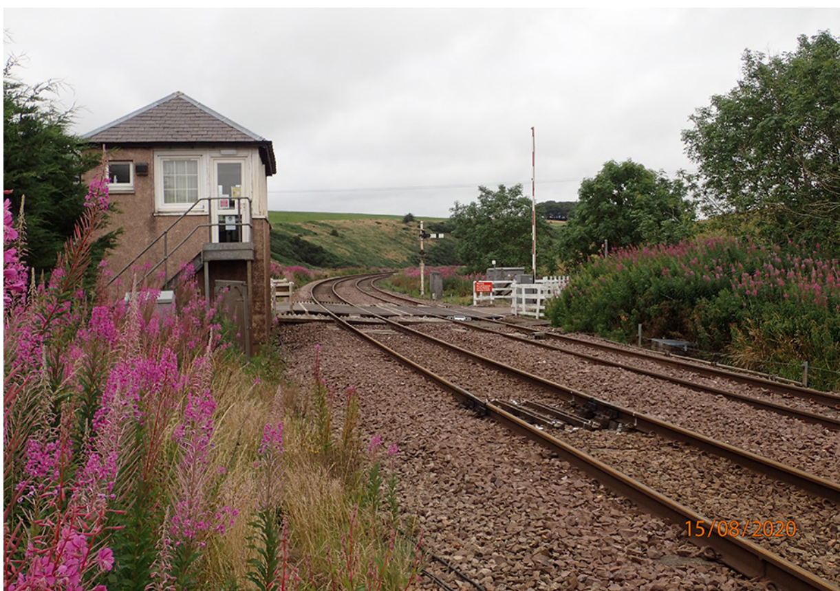
Figure 57: Carmont signal box looking north
