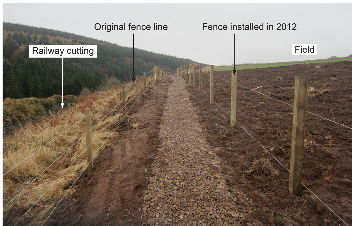
Figure 45: Drain shortly after completion in late 2012 showing section between CP11 and CP16 looking south (Network Rail)
