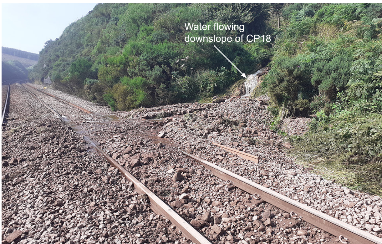
Figure 19: Washout debris on the track approximately 55 minutes after the accident. A short length of scrap rail unrelated to the accident is also visible (Story Contracting)
