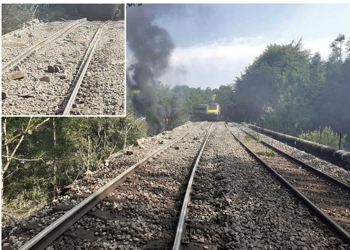
Figure F.2: Track damage across bridge 325 at 10:35 hrs on 12 August 2020 (Story Contracting)
