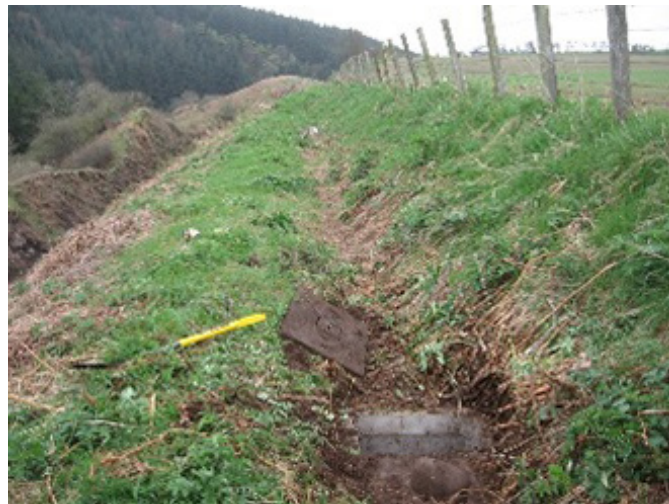
Figure G.1: Pre-2010 crest drain catchpit between CP10 and CP16 showing drain close to the cutting crest in 2010 (Carillion)
