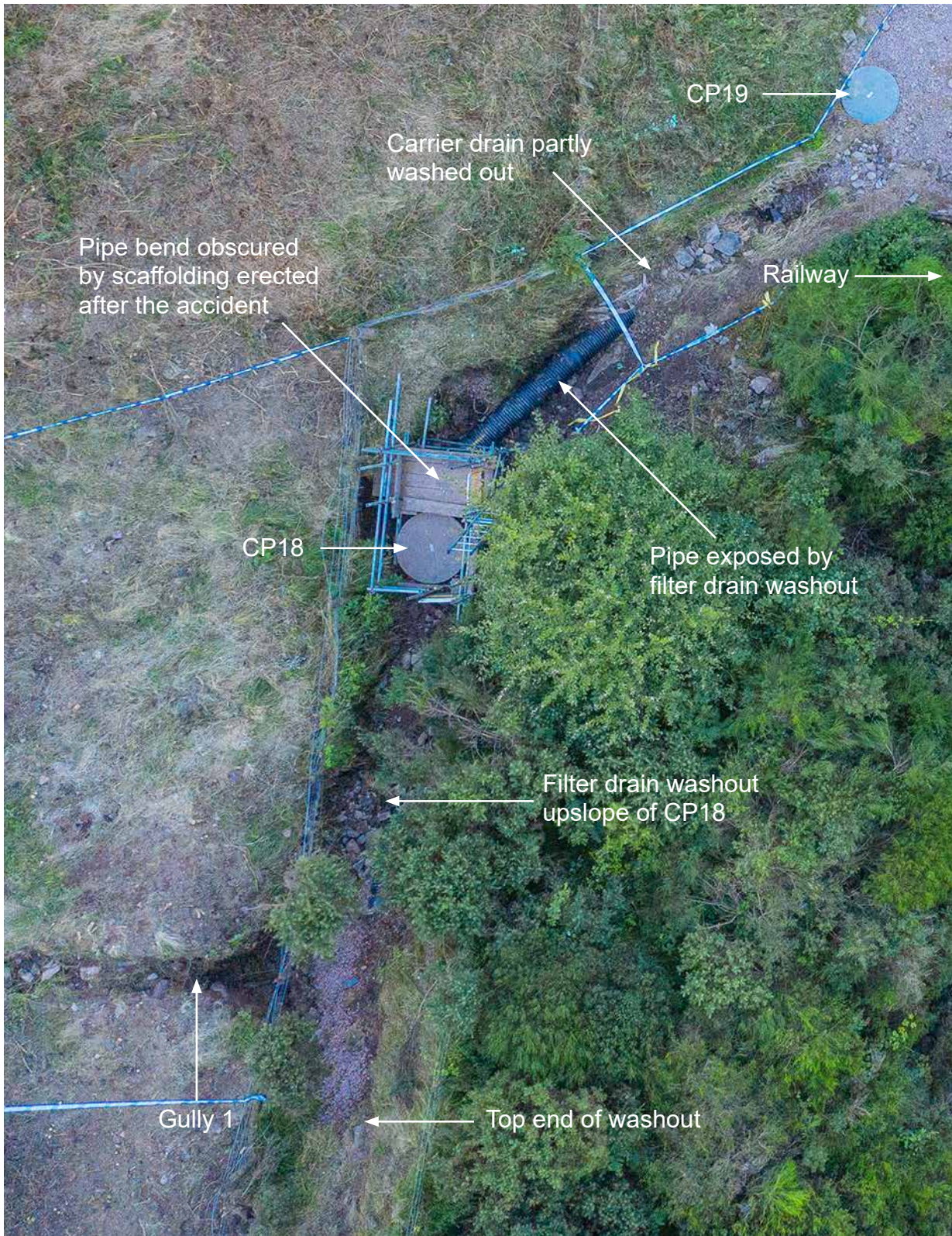
Figure 17: Aerial view of CP18 showing extent of washout (Scan Station/Network Rail)
