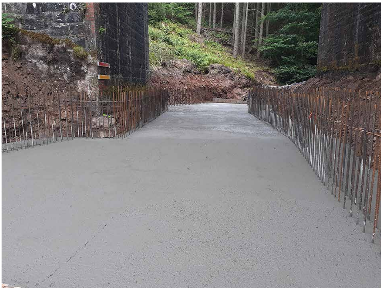
Figure F.10: Scour protection works at bridge 325 on 11 August 2020 (Story Contracting)
