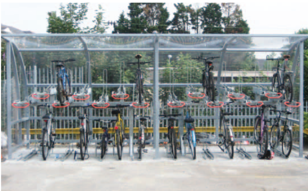
Two tier racks within covered cycle shelter
