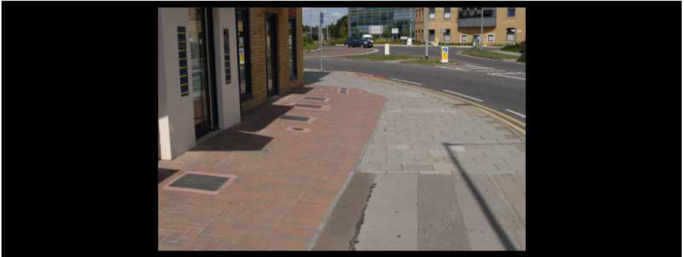
What not to do: plot demarcation ignoring the existing footway creates a disjointed public realm
