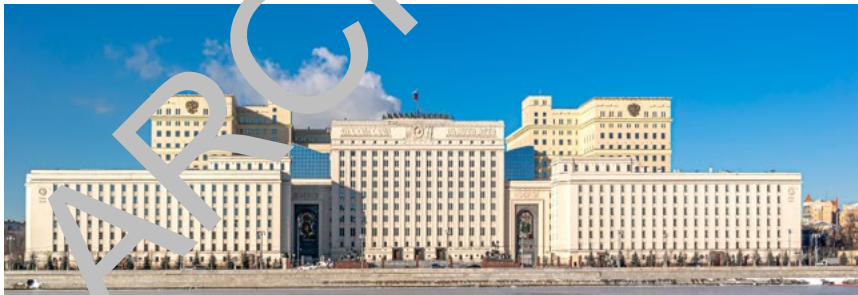
The National Defense Management Center of the Russian Federation coordinates the activities of all ministries in the interests of ensuring the defence of, and security of, the state
