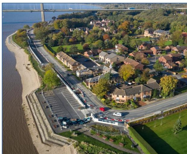
The Hesse Foreshore Tidal Defence Scheme is an East Riding of Yorkshire Council project which included the construction of a 465-metre long, 1m-high glass and concrete wall along Cliff Road, Hesse, to help shield the area from flooding caused by tidal surges along the Humber.
