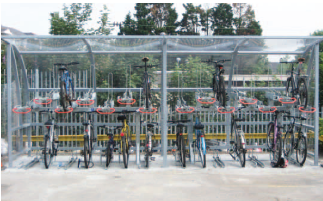
Two tier racks within covered cycle shelter
