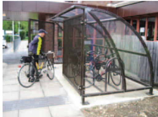
Covered shelter secured with lockable gates
