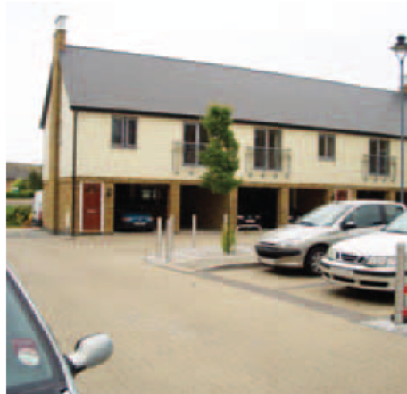
Undercroft parking facing onto central parking court
