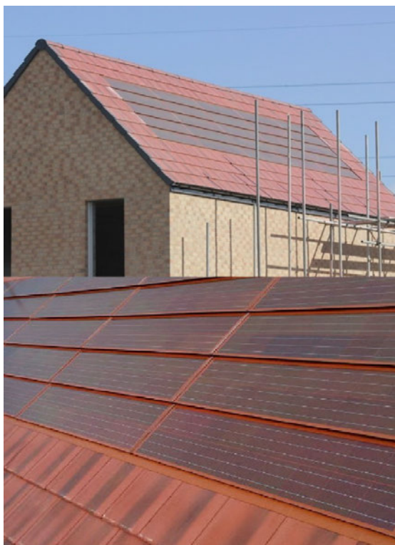
Integrated photovoltaic clay-type roof tile (source: Romag)
