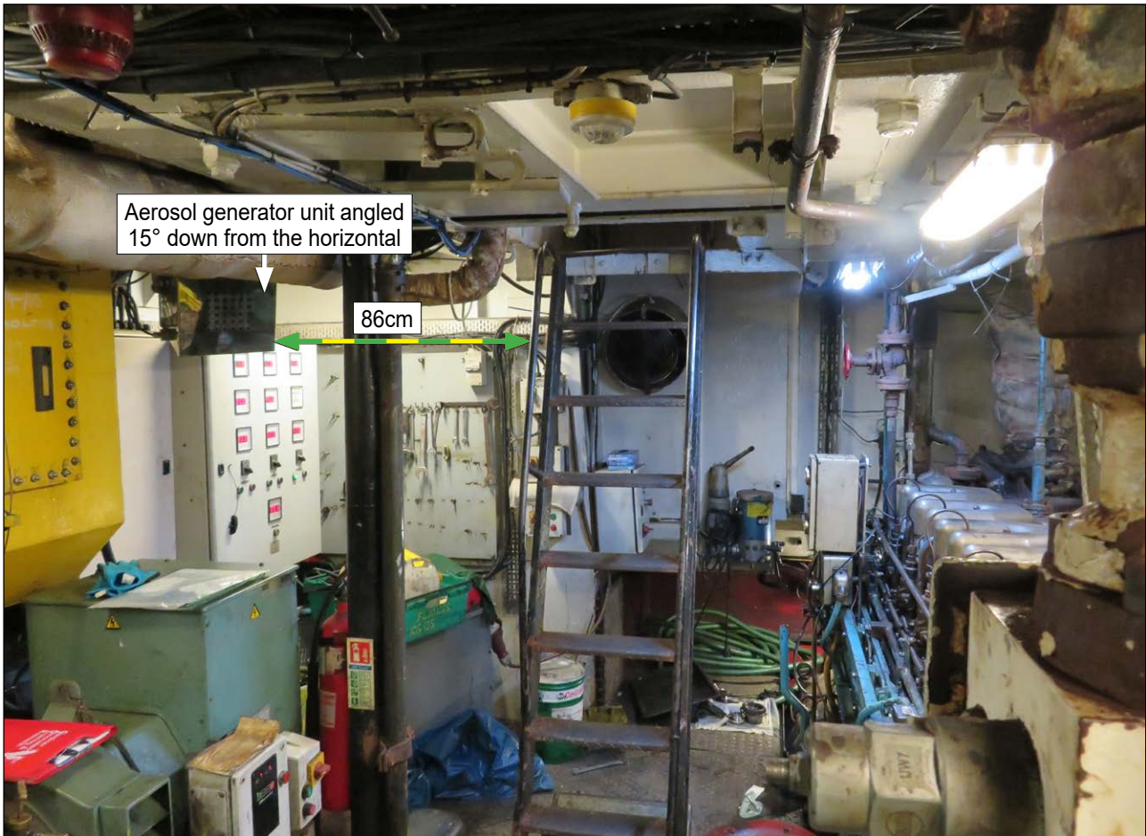
Figure 9: View of engine room looking aft, showing position of aerosol generator unit adjacent to the access ladder
