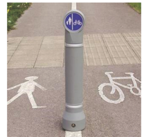
Figure 1. Typical bollard to be provided at key intersections, and to either end of cycle routes to demarcate suitable side of use for cycles and pedestrians.
