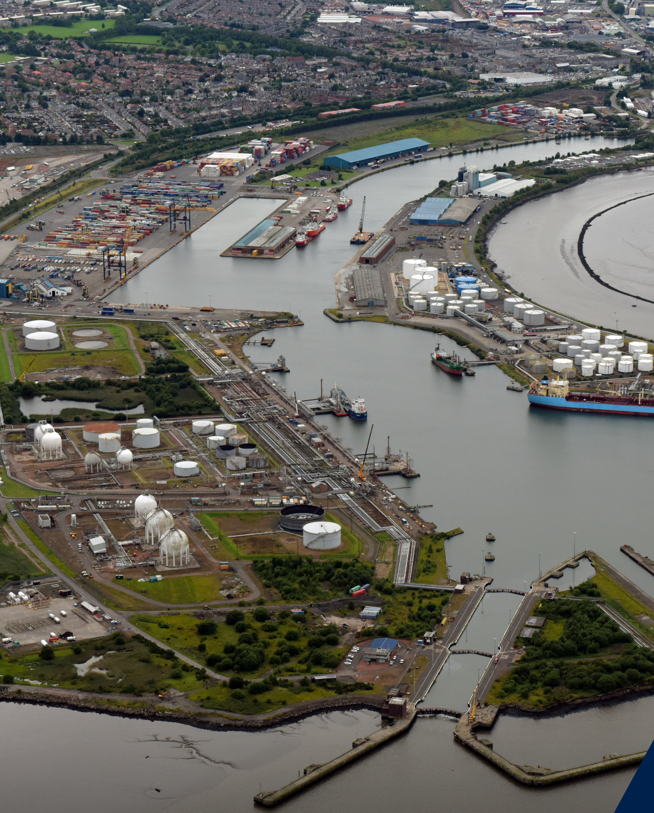
Aerial view of Grangemouth port facility. Photograph reproduced with permission from INEOS. © INEOS Limited 2016 all rights reserved.
