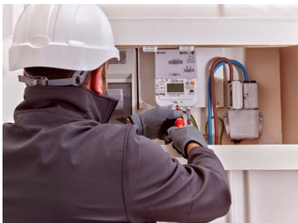
Figure 7: A smart meter being installed
