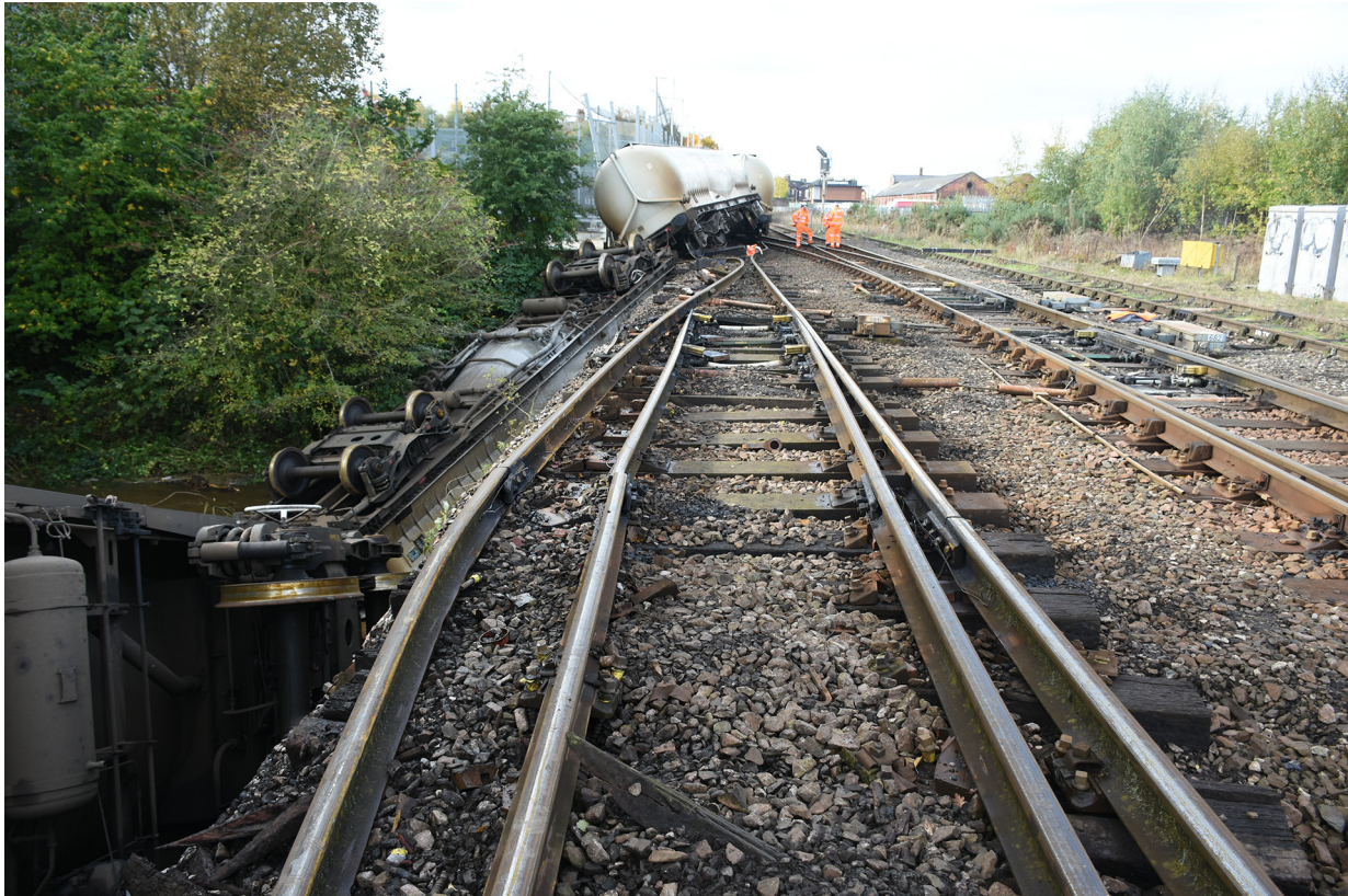
Figure 20: Damage to the track and bridge at Petteril Bridge Junction.
