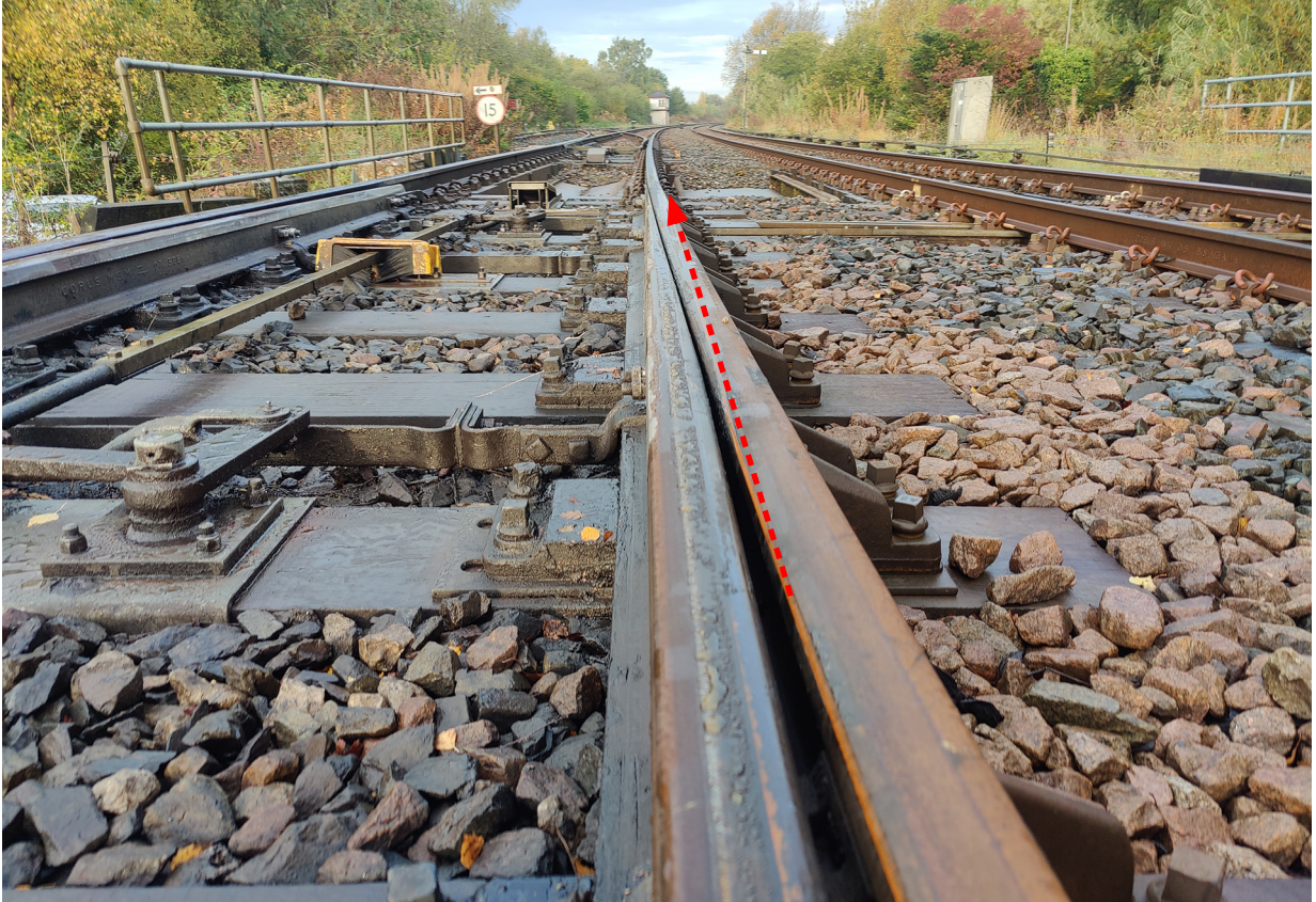
Figure 29: False flange marks at Howe & Co's Siding.
