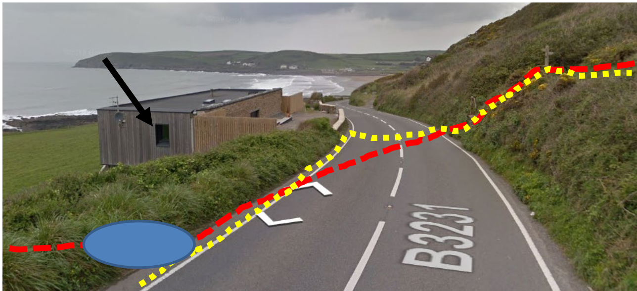
iii). Oyster Falls (black arrow) – current SWCP – yellow dots, proposed ECP - red dashes. Pedestrian refuge – blue area.
