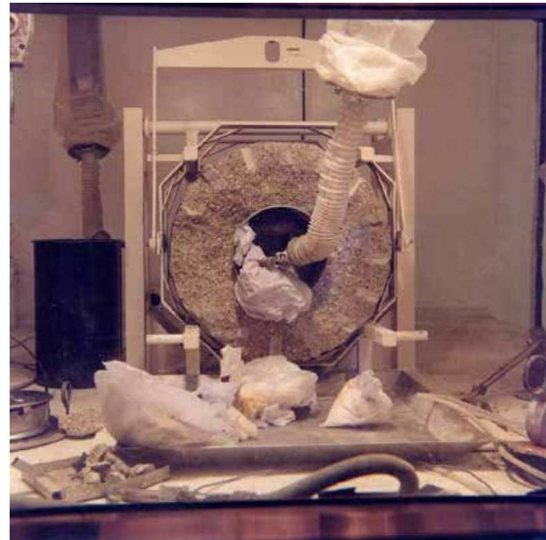
Repacking a concrete lined drum
