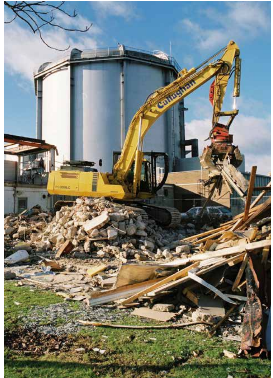
Demolition work at Harwell
