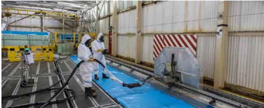
Decontamination work inside the Dounreay Materials Test Reactor
