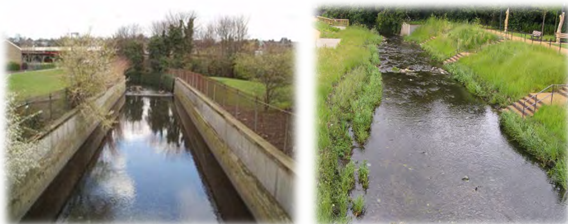
Figure 10-3 Example of Enhancement. River restoration as part of the 'Urban Renaissance in Lewisham' programme. The lefthand picture shows the river before restoration, the righthand picture is after enhancement. Restoration action included removing the concrete walls, regrading banks, improving riparian habitat and marginal planting, and installing gravels in the river channel.
