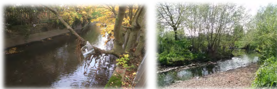
Figure 10-4 Example of Enhancement. Tokynton Park, River Brent River Restoration Project. The lefthand picture shows the river before restoration, the righthand picture is after enhancement. Restoration action included re-meandering channels, reinstating varied flow types and in channel features. Hard revetment was removed and banks reprofiled.
