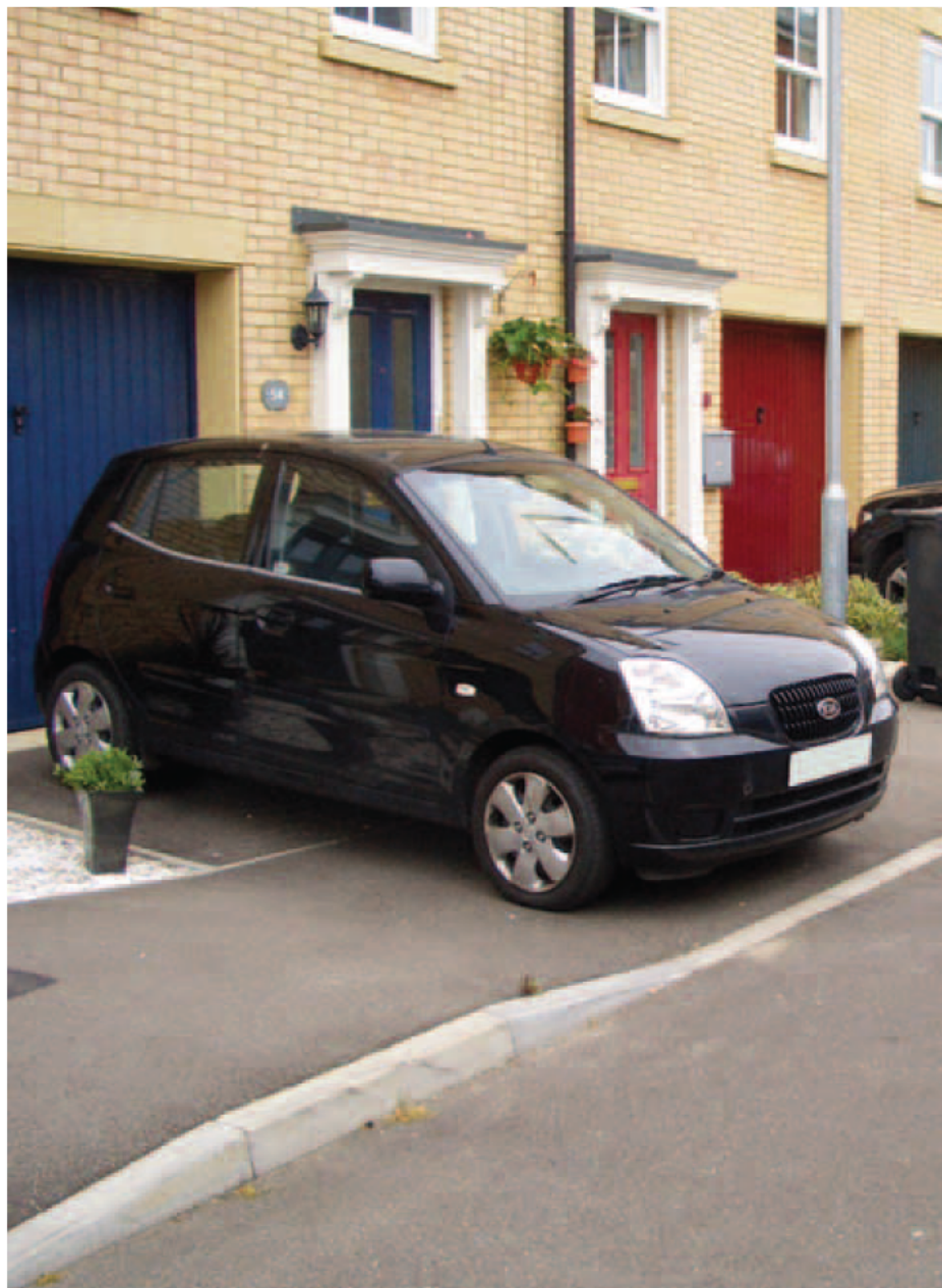
Setbacks from garages and gates lead to vehicles parking in front of garages and blocking footways
