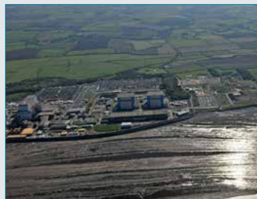
Hinkley Point A and the EDF owned (B) station
