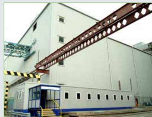
Magnox Reprocessing Plant
