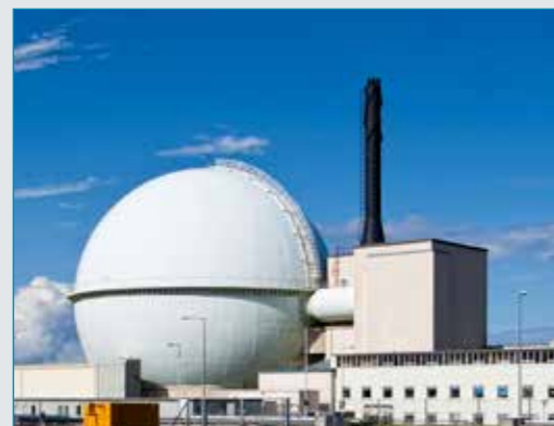
Dounreay Fast Reactor
