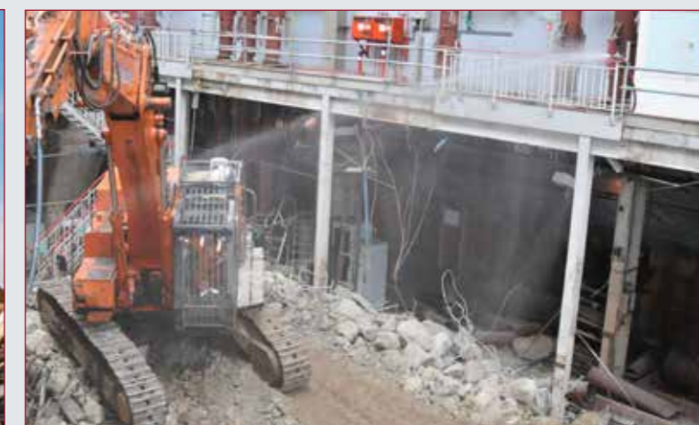
Turbine hall demolitions
