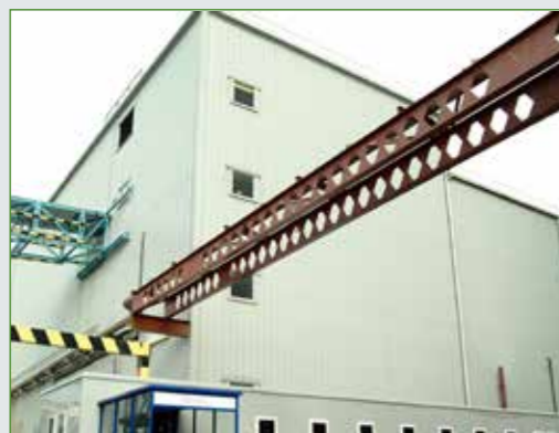
Magnox Reprocessing Plant
