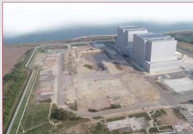
Bradwell in care and maintenance
