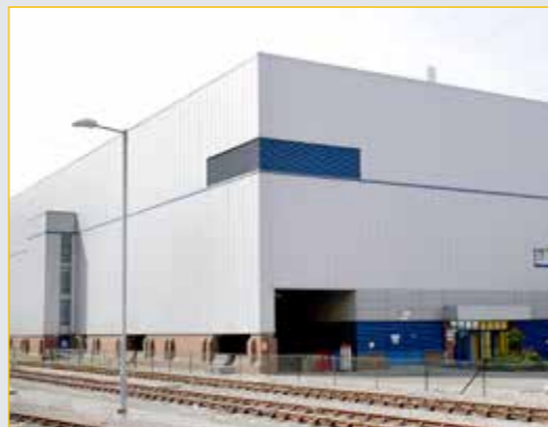
ILW Treatment and Storage at Sellafield
