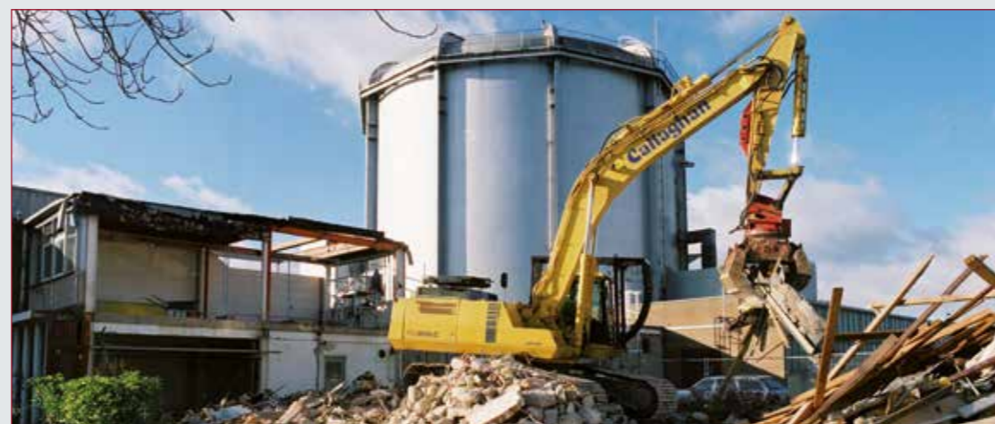
Demolition work at Harwell
