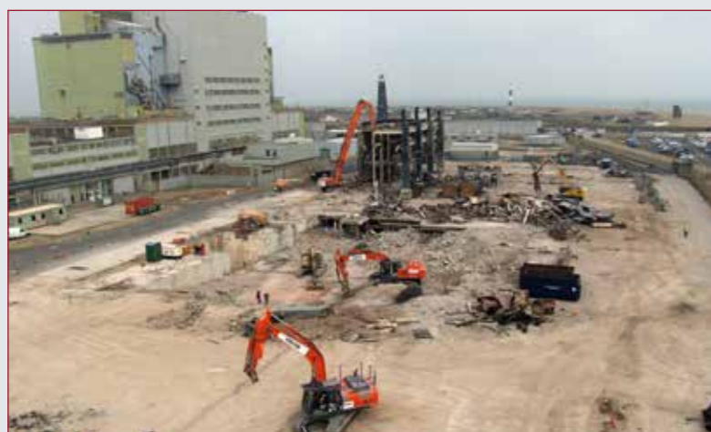
Demolition work at Dungeness
