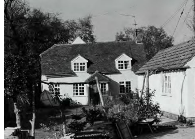
Figure 13 Beech Cottage 1975 (© Historic England)
