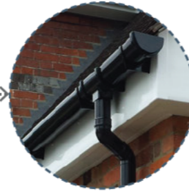
BLACK UPVC GUTTERING
