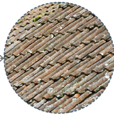
CONCRETE ROOF TILES
