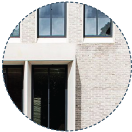
RENDER AND BRICKWORK
