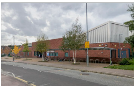
13 TAKELEY PRIMARY SCHOOL
